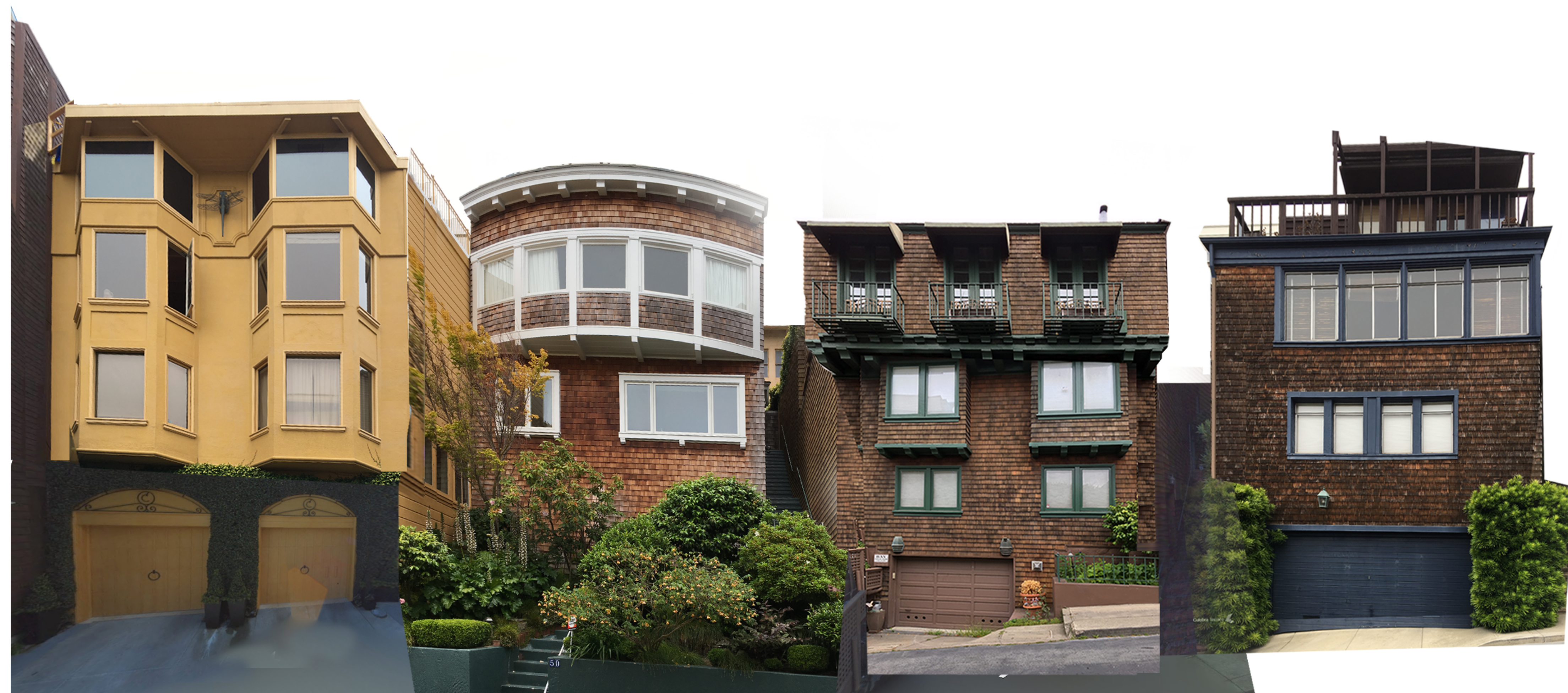
BUILDINGS OPPOSITE OF PROJECT SITE
