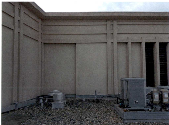
Sector A- Antenna location
