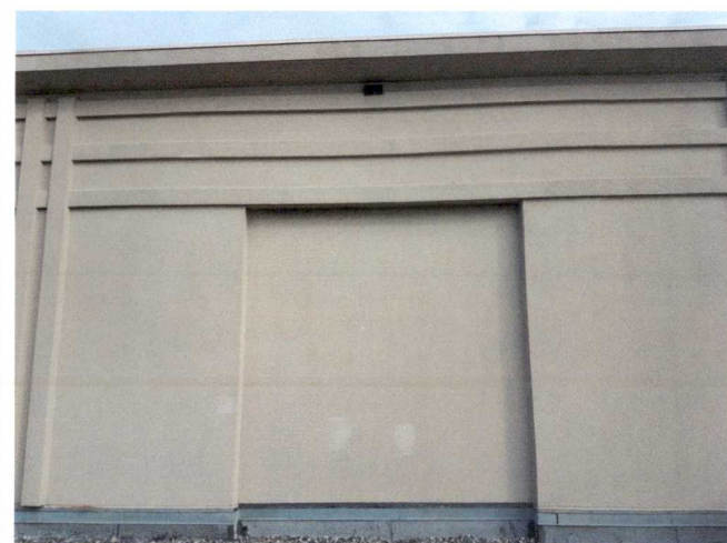
Sector C- Antenna location
