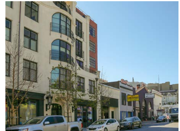
Setting back the portion adjacent to the neighboring building helps ease the change of scale.
