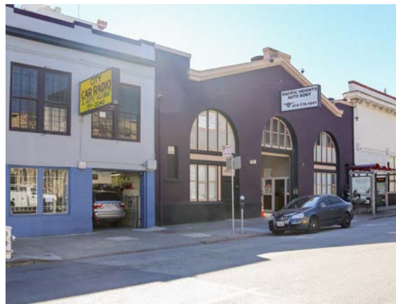
Look for ways to preserve old buildings for new uses in meaningful ways.
