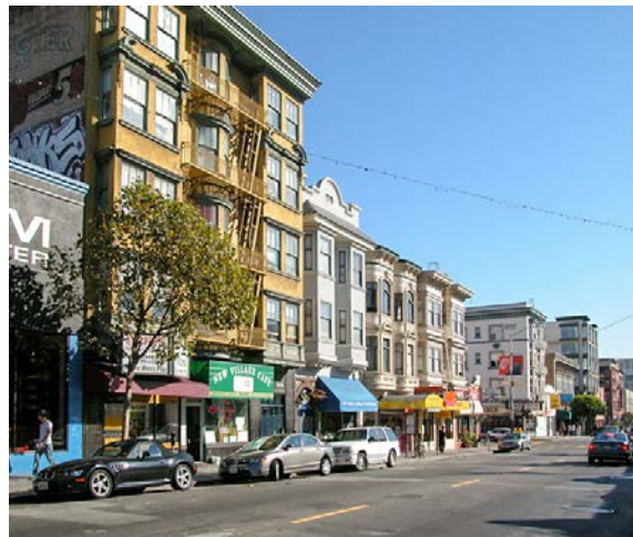
Vertically proportioned windows with divided lites reflect the prevailing scale of the neighborhood.
