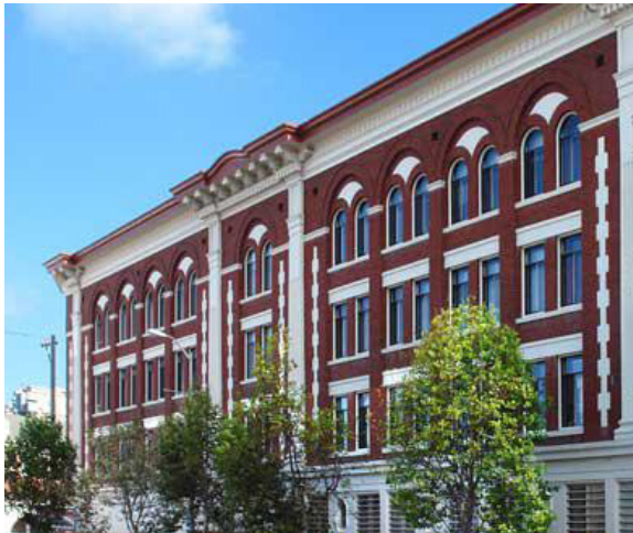
A facade is modulated with the spacing pattern of windows.
