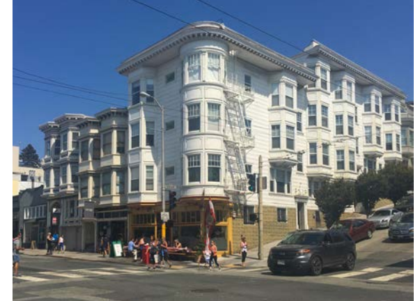
This building reinforces the streetwall by stepping with topography which also modulates its scale.
