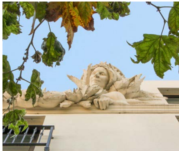
The spirit of artistic detail of this building give it life and a unique identity, but it also shares common materials and features with its neighbors.
