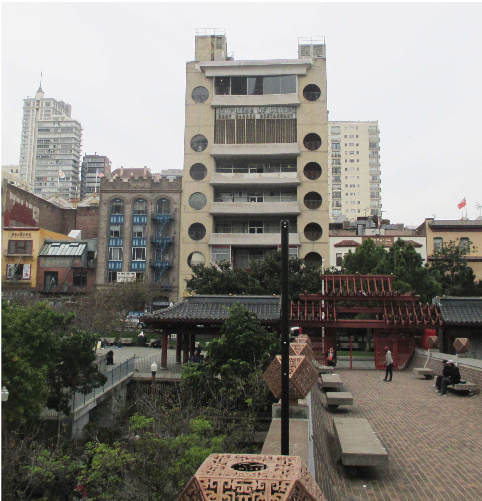
REAR FACADE & PORTSMOUTH SQUARE
