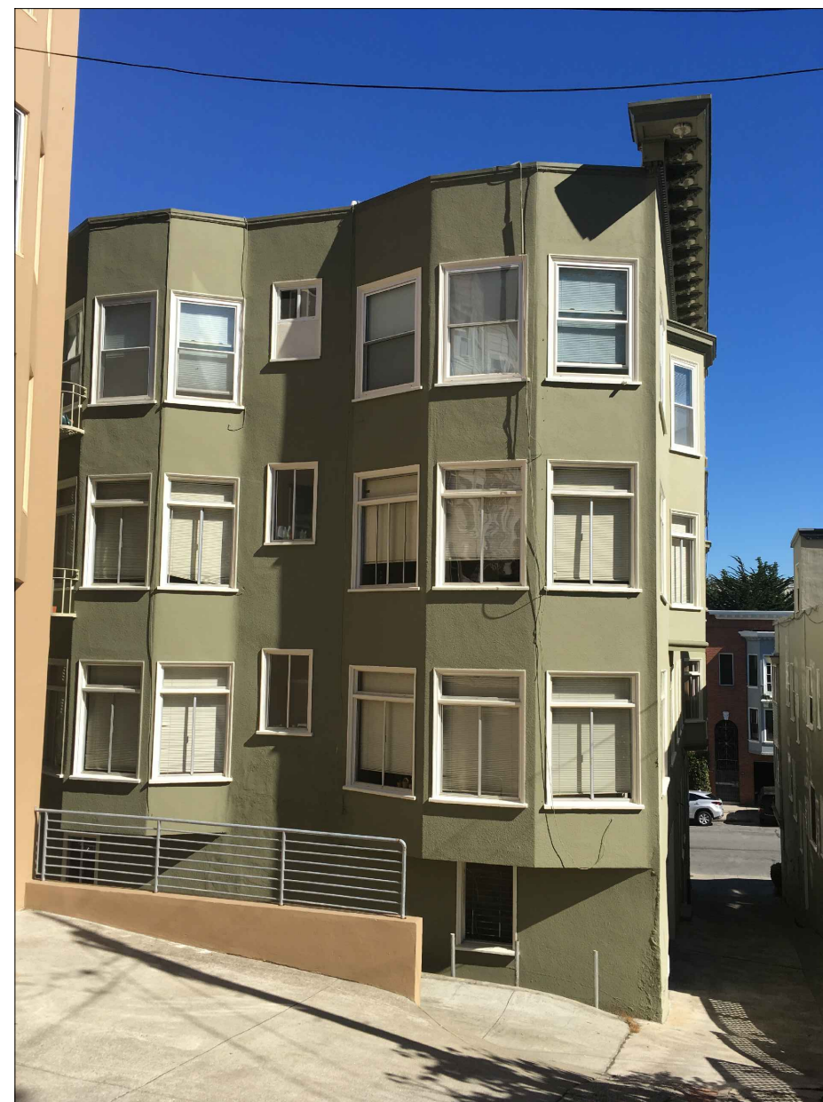
4 REAR OF ADJACENT BUILDING
