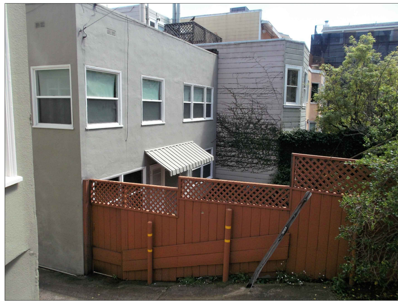
3 REAR FACADE AND ADJACENT BUILDING
