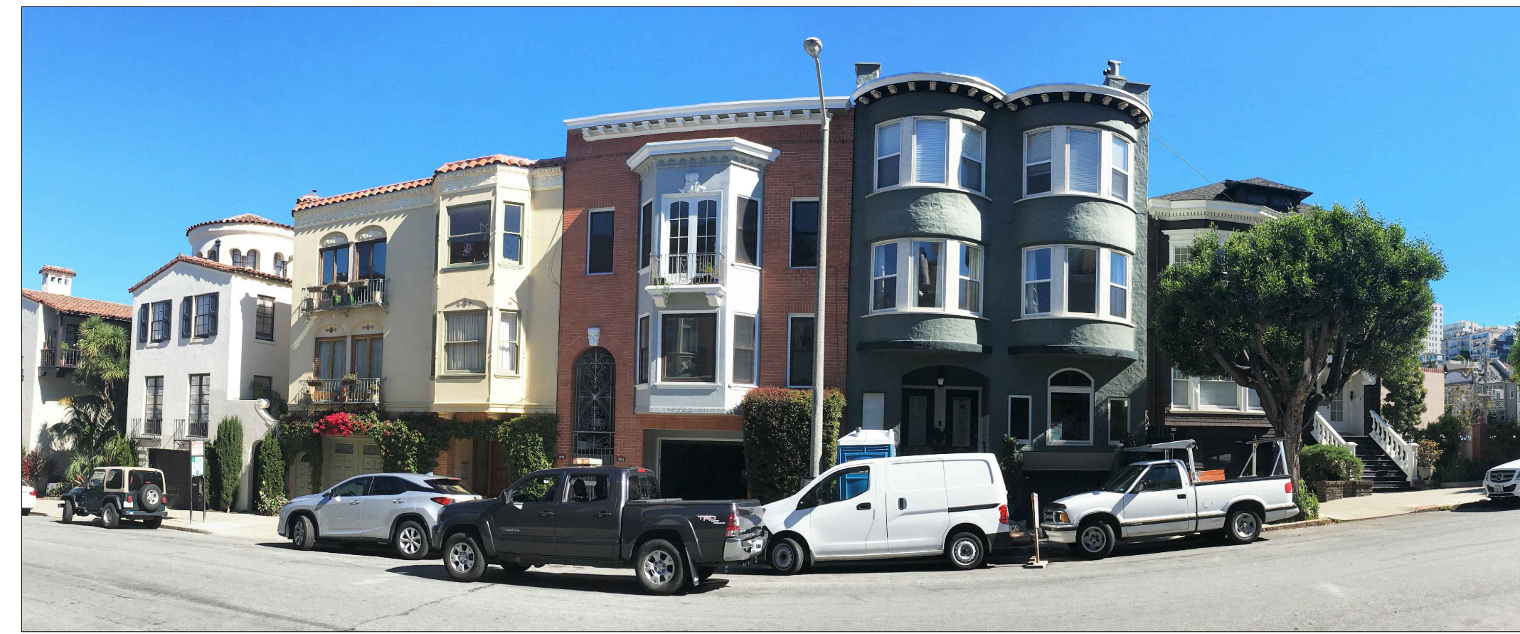
2 BUILDINGS ON OPPOSITE SIDE OF STREET
