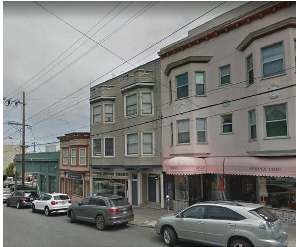
01 - VIEW ALONG FILLMORE STREET
