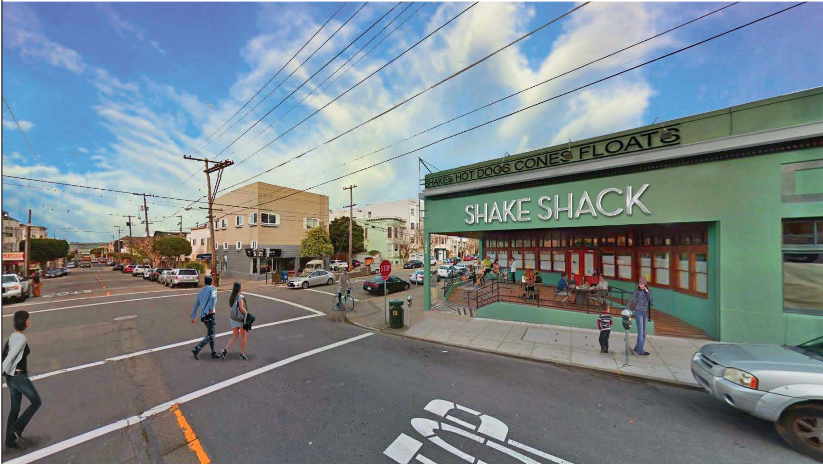
EXTERIOR VIEW - SHAKE SHACK
