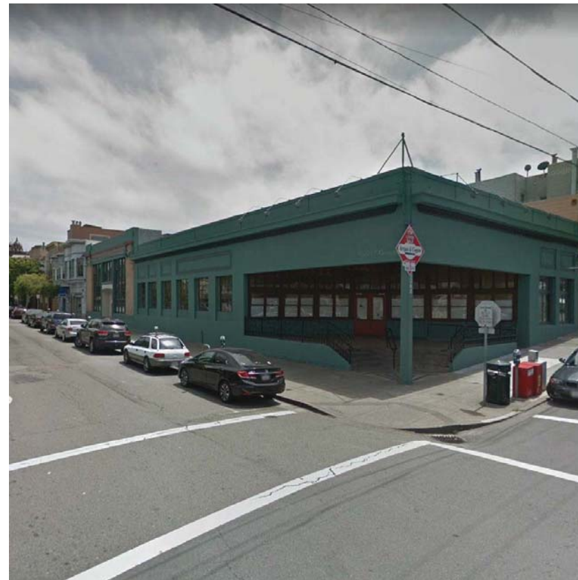
04 - VIEW ALONG FILBERT STREET
