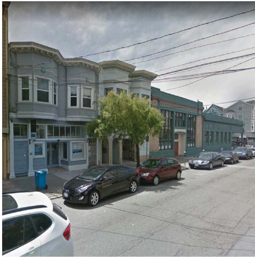
03 - VIEW ALONG FILBERT STREET
