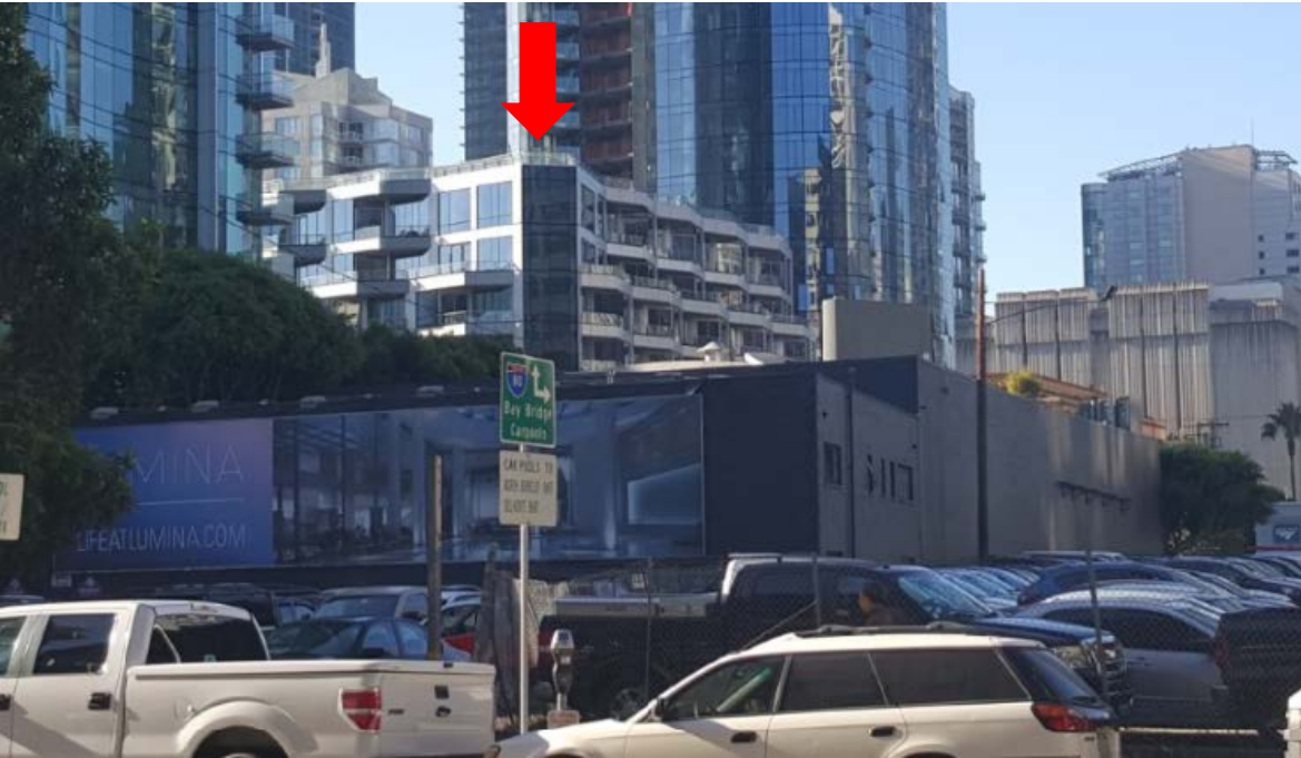
View of Building from Spear Street facing Southwest
