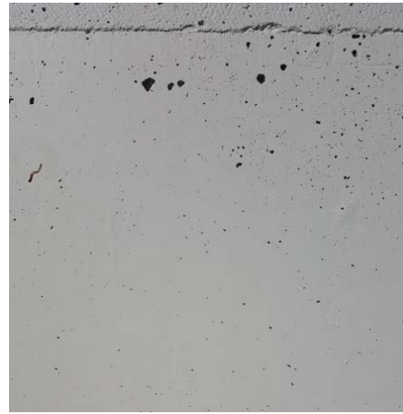
Close up of Penthouse wall
