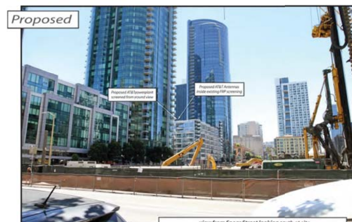
view from Spear Street looking south at site AdvanceSim PHOTO SIMULATION SOLUTIONS Contact: (925) 360-8107 AT&T Wireless CCL04727 Podium Building A at 318 Main-Perm 318 Main Street, San Francisco, CA Photosims Produced on 8-7-2017
