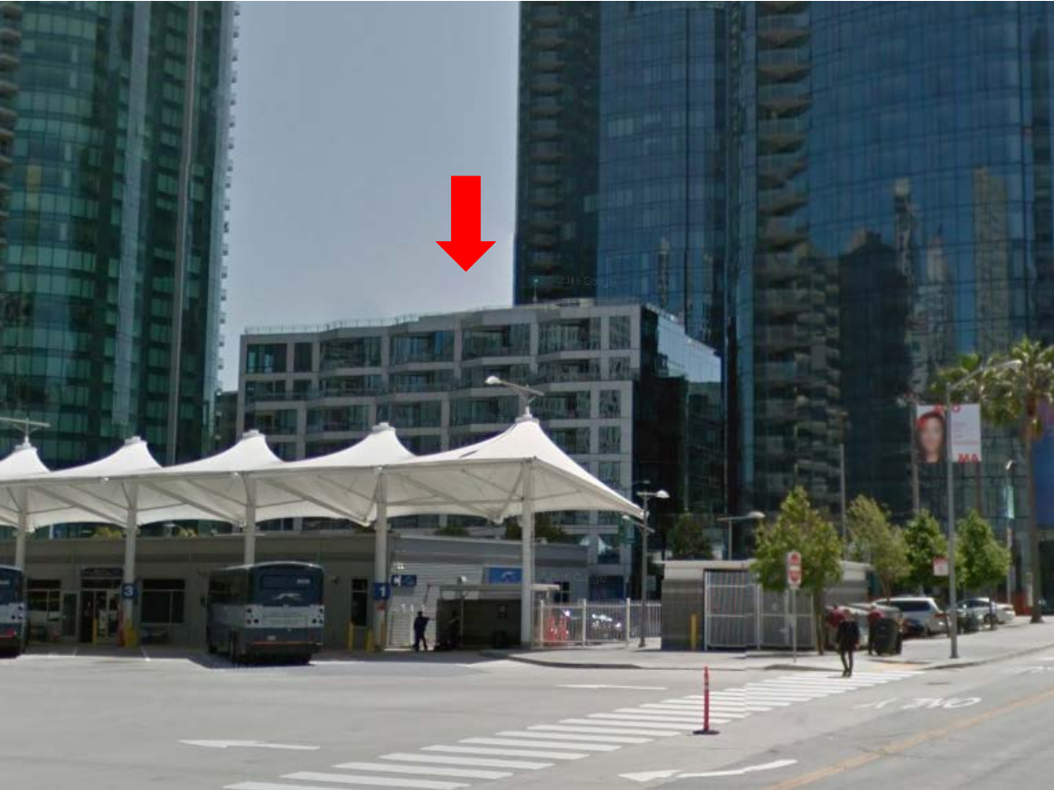
View of Building from Beale Facing East
