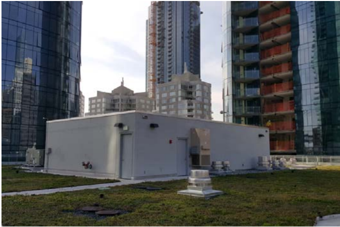
Close up of Rooftop Penthouse
