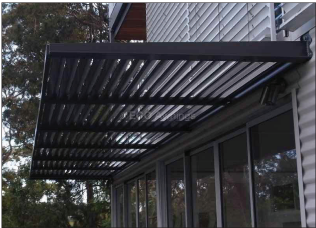
SHADE STRUCTURE TRELLIS AT BUILDING CORNICE. BRONZE COLOR TO MATCH WINDOW FRAMES. ⑦
