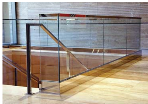
13 GLASS GUARDRAIL REFERENCE "B" 6" = 1'-0"
