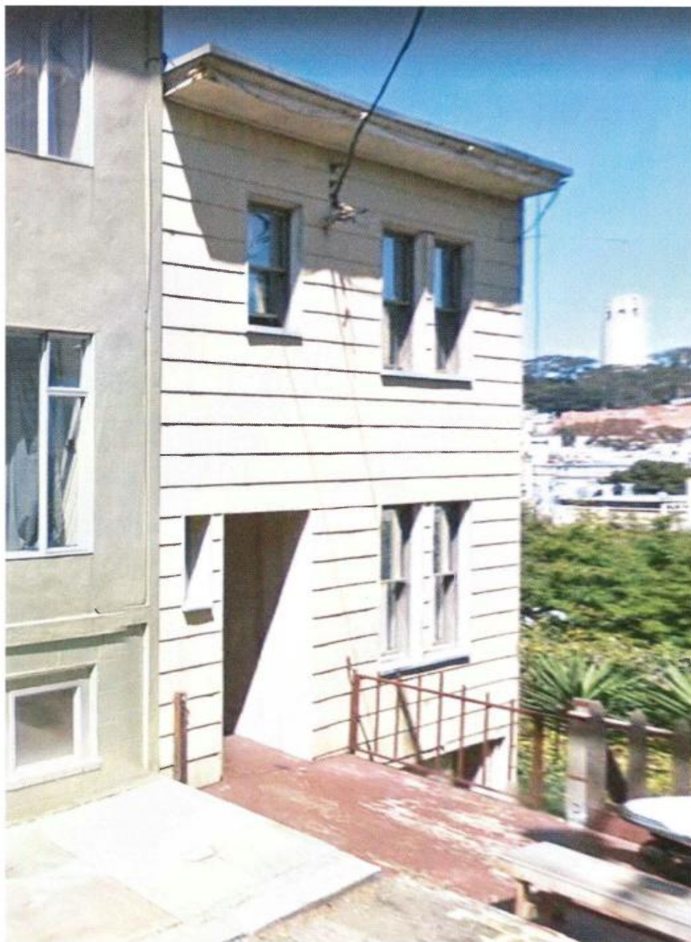
10-12 Aladdin Terrace, primary façade (Google street view image)
