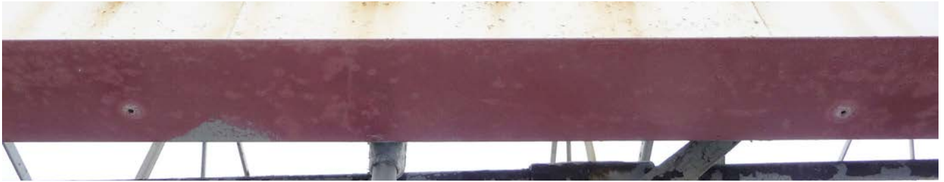
Figure 5 - Weep holes are drilled into the base of the letters. They exist in various conditions as shown in the three images below.
