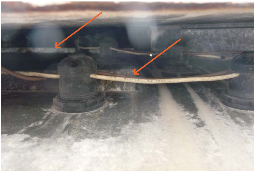
Figure 22 - Interior supports installed for stability are evident on the front face of the letter.
