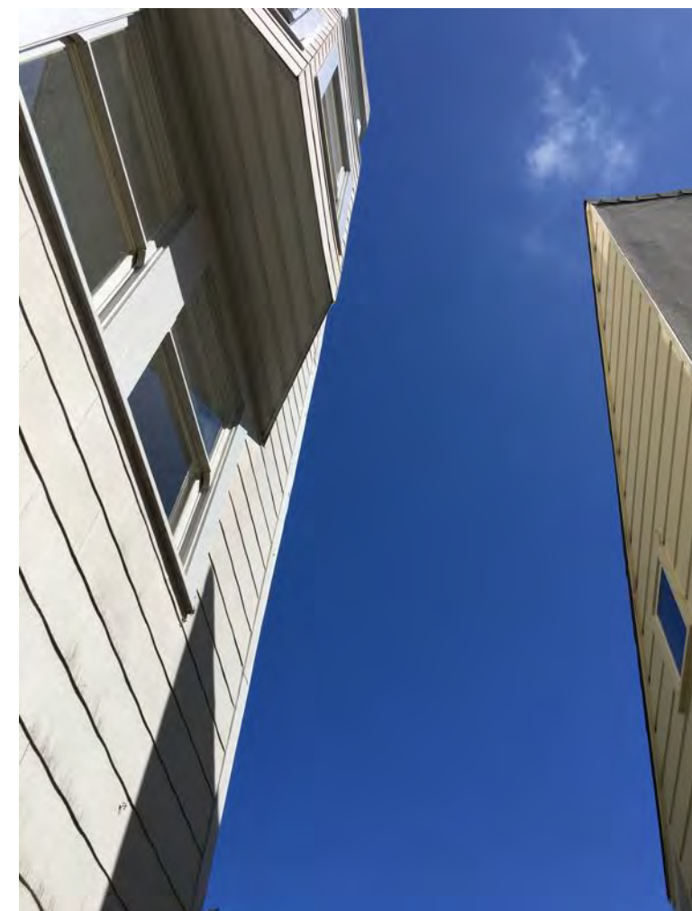
SUBJECT PROPERTY: 50 SEWARD ST.: REAR
