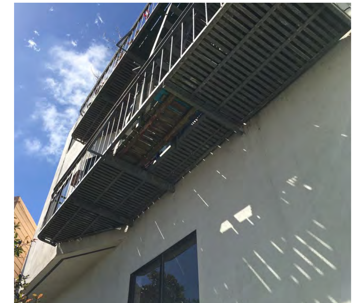
ADJACENT PROPERTY: 998 SANCHEZ STREET: REAR
