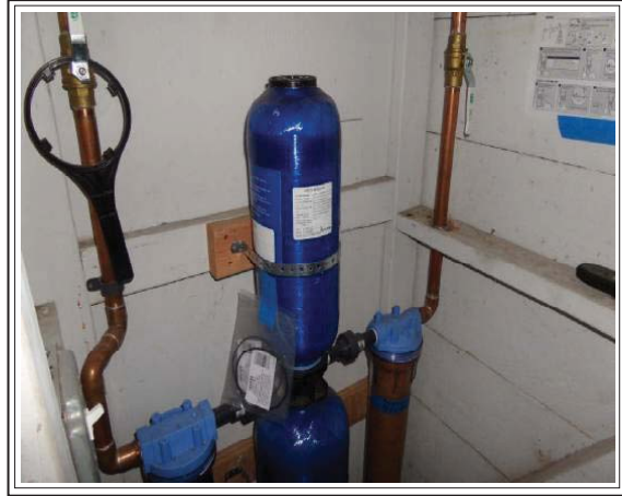
View of Existing Water Filtration System
