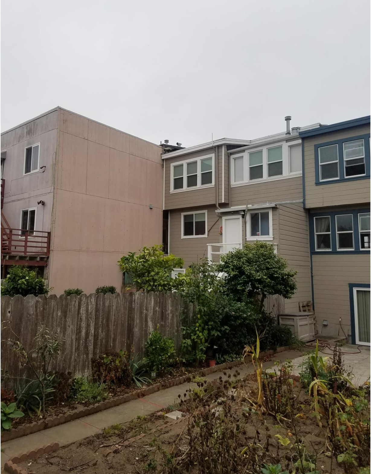
*View the single-family home directly west of the project site at 2420 Tarval Street.
