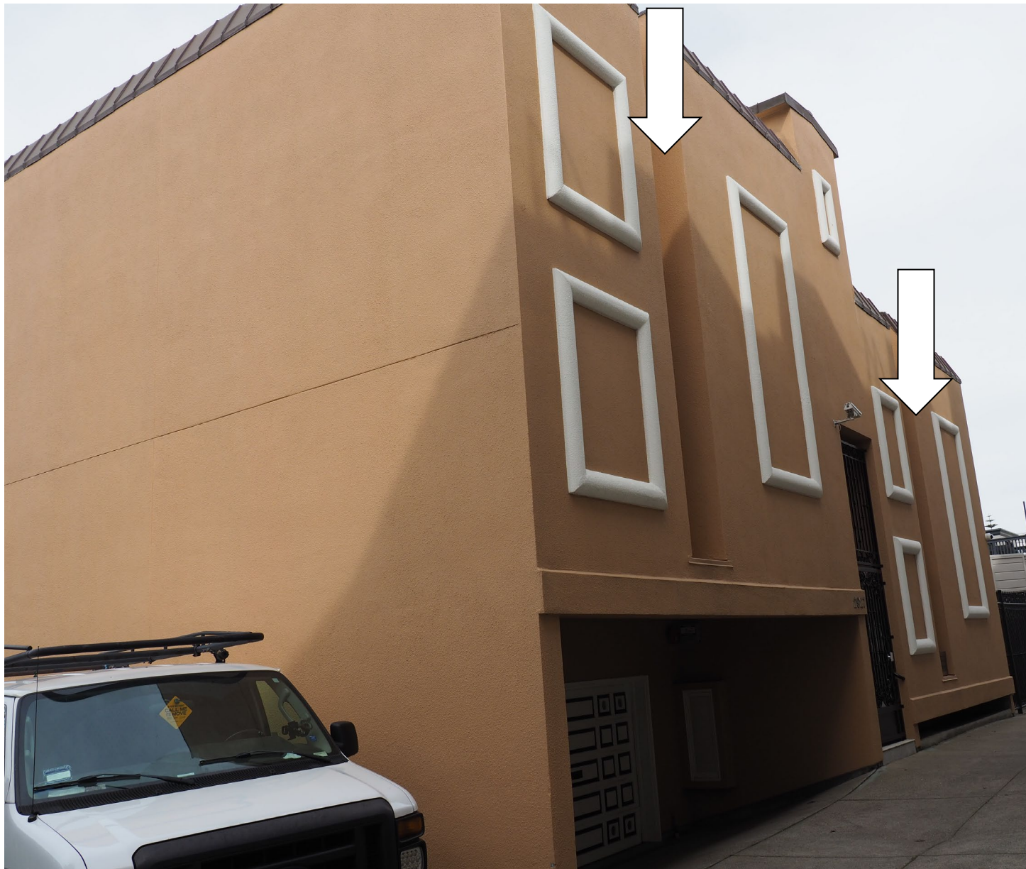
Figure 1. South Elevation of 2927 Larkin Street – Arrows indicate location of narrow inset windows that provide limited light to two bathrooms, an office and kitchen.
