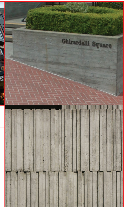
BOARD FORMED CONCRETE
