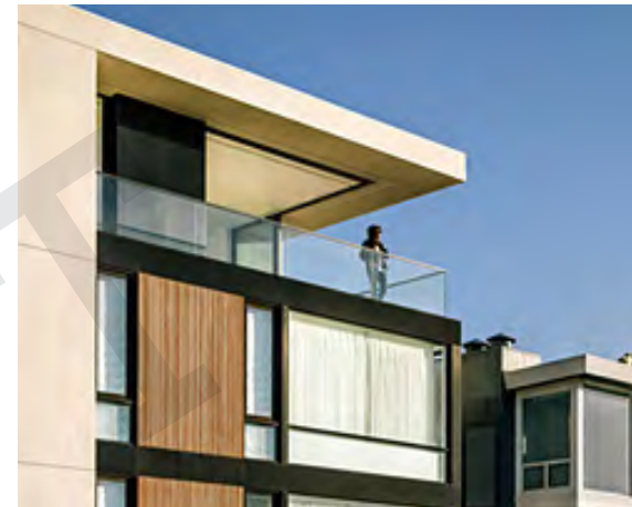
Building tops can connect inside and outside spaces.
