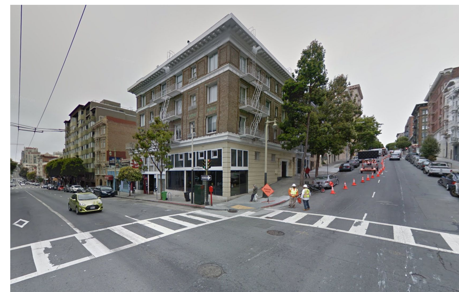
POST STREET VIEW FROM THE EAST
