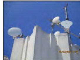
22. Microphone Antennas on Southwest side of Perthouse
