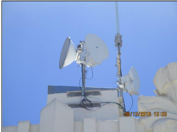
19. Microwave and Omni Antennas on Northeast side of Penthouse
