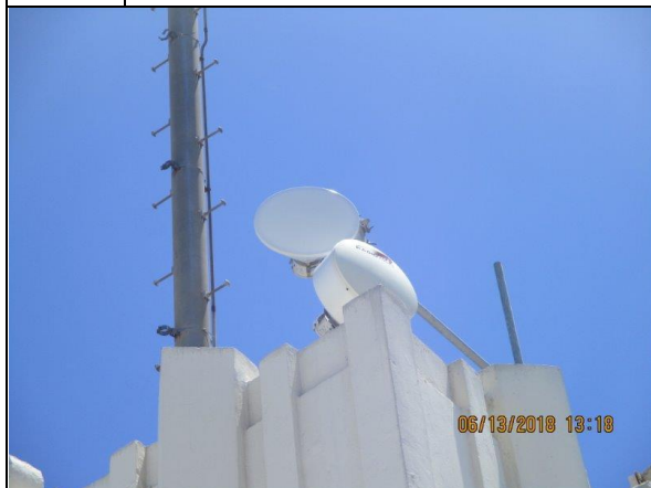
20. Microwave Antennas on Northwest side of Penthouse
