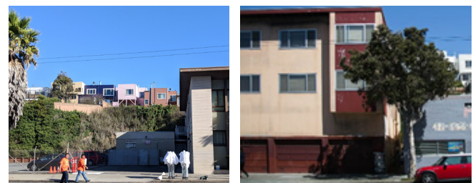
INACTIVE FRONTAGES ALONG MISSION STREET
