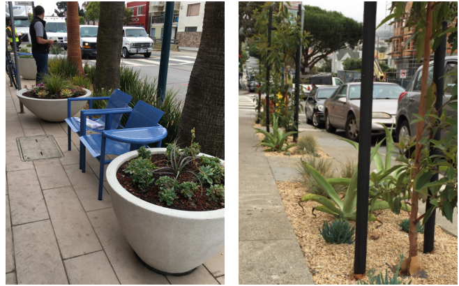
OCEAN AVENUE STREETScape IMPROVEMENTS ACCORDING TO THE OCEAN AVENUE CORRIDOR DESIGN PLAN ( HTTPS://SF-PLANNING.ORG/OCEAN-AVENUE-CORRIDOR-DESIGN )
