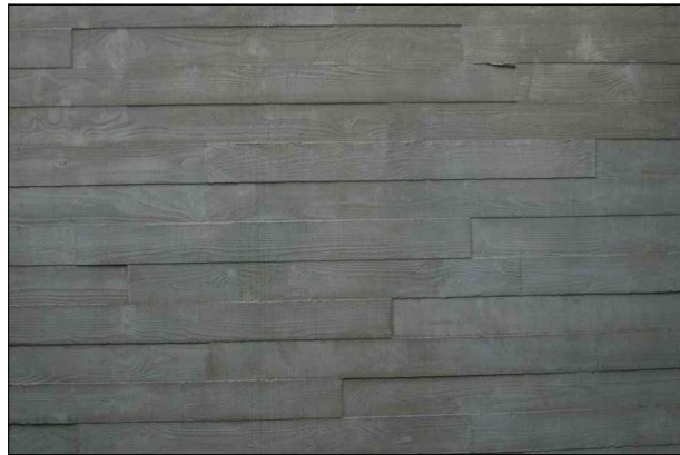
Board formed concrete
