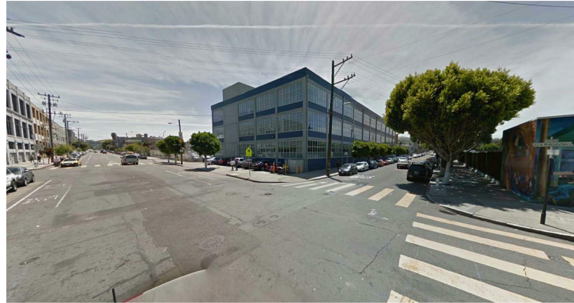
2. VIEW FROM TREAT AVE LOOKING EAST
