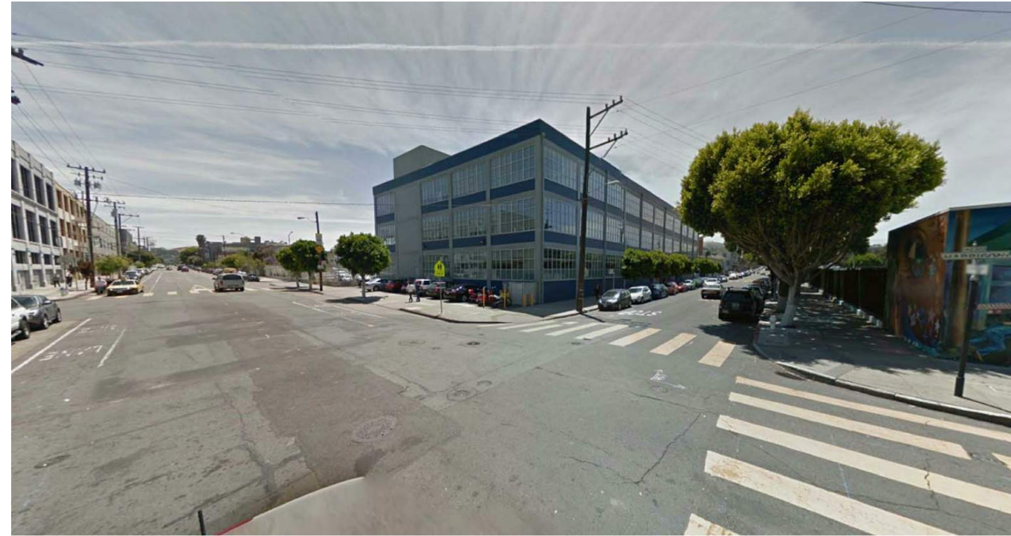
2. VIEW FROM TREAT AVE LOOKING EAST
