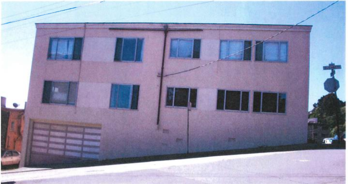
Secondary façade facing north
