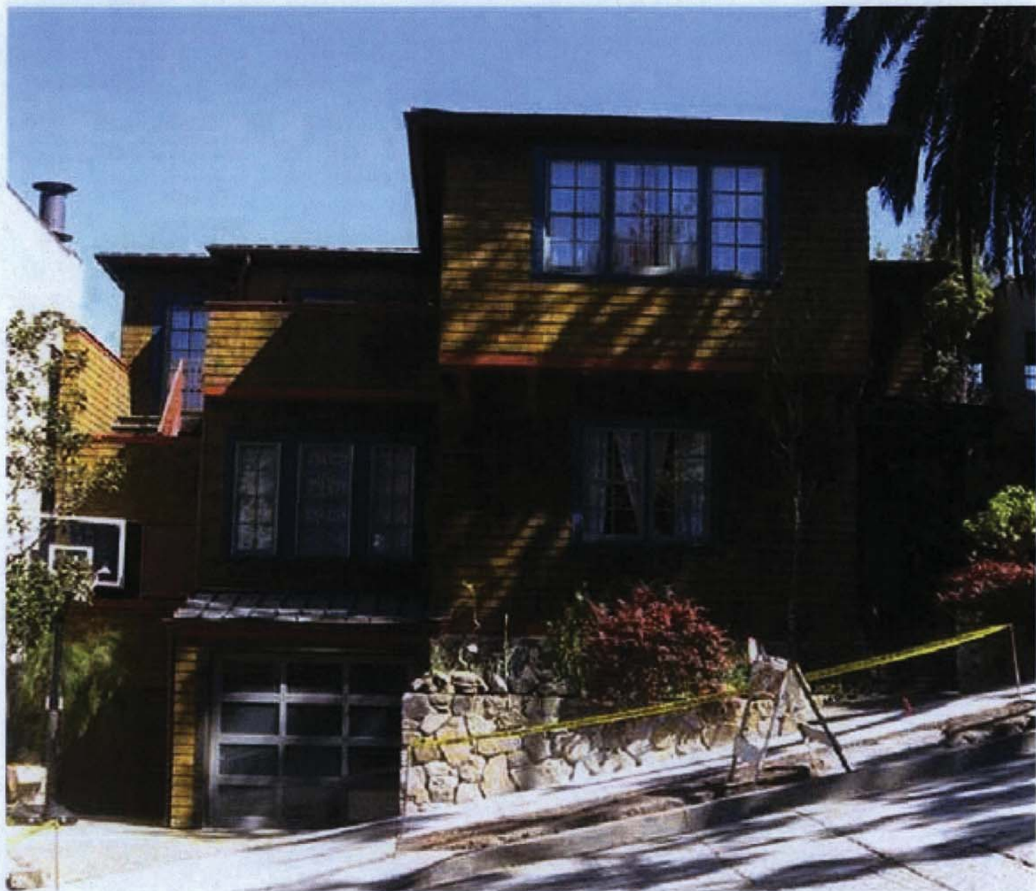
Existing Building at 775-77 Sanchez Street
