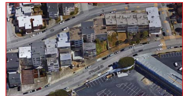
Existing Conditions on South Side of O'Farrell St. (Opposite City Center)
