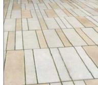
PERMEABLE CONCRETE PAVER LABYRINTH PATTERN
