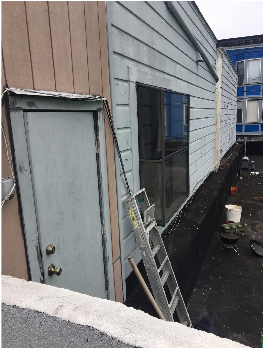
View of Existing Property Line Door and Window
