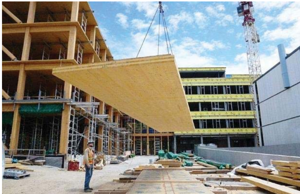
Installation of a cross-laminated timber panel on-site
