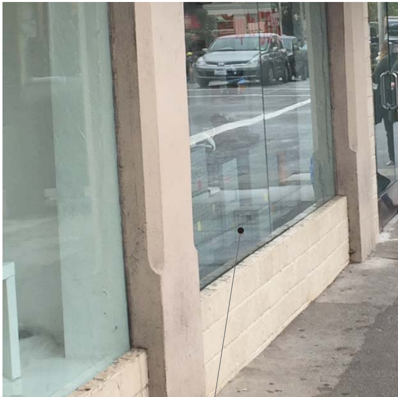
Existing storefront frameless window system with center butt joint glass
