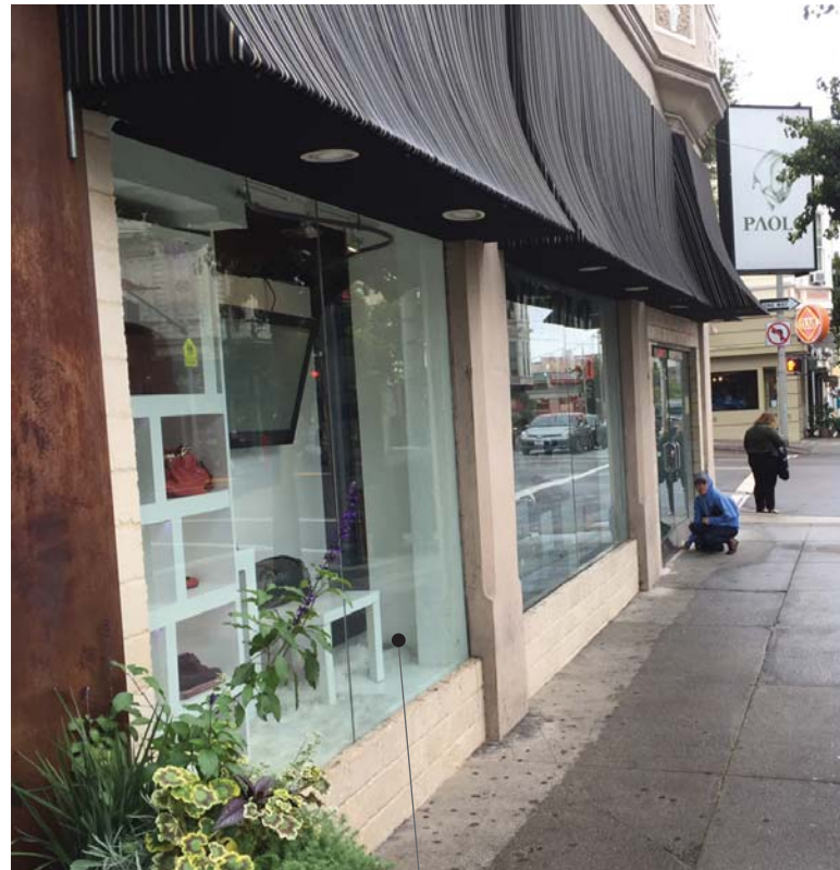
Existing storefront frameless window system with center butt joint glass
