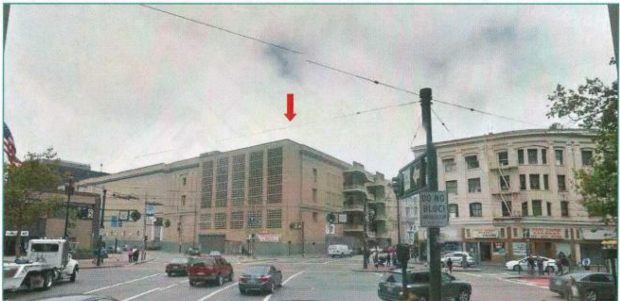
View of site looking North West on Market Street
