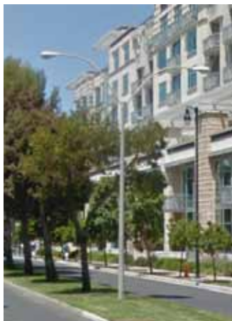
Existing Street Light Type 2
