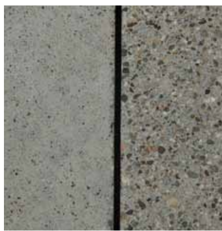
Concrete Paving at Sidewalk
