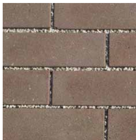
Unit Paving in Planter Strip
