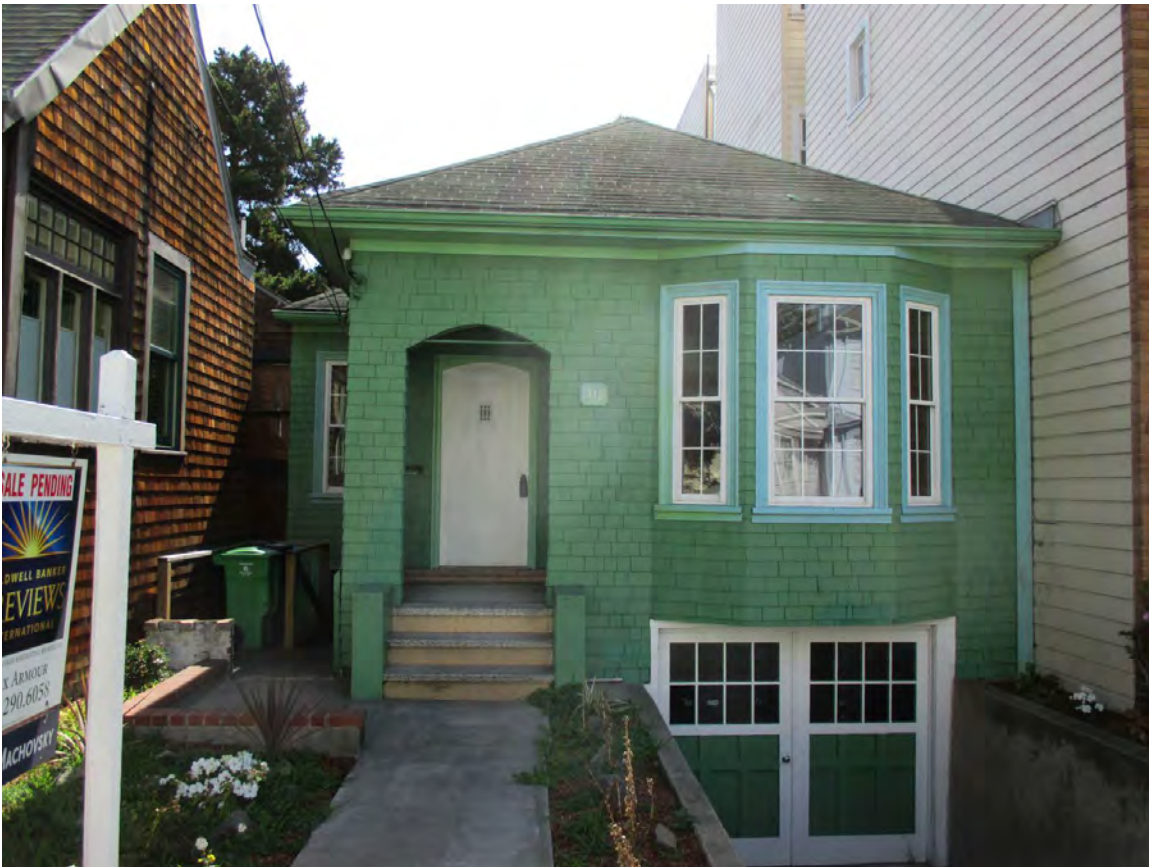
Figure 14. Primary façade, looking east Source: Christopher VerPlanck
