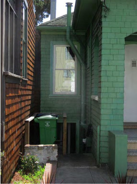
Figure 15. Lightwell, looking east Source: Christopher VerPlanck
