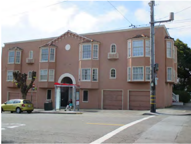
Figure 4. 6743-49 California Street, looking south Source: Christopher VerPlanck
