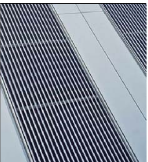
7 TRANSLUCENT VENTILATING LOUVER
