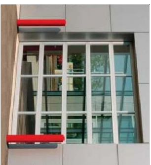
10 OVERHEAD GARAGE DOORS
