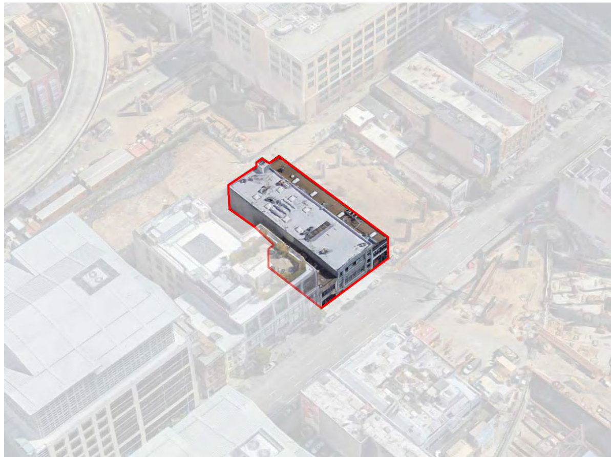
View from North
