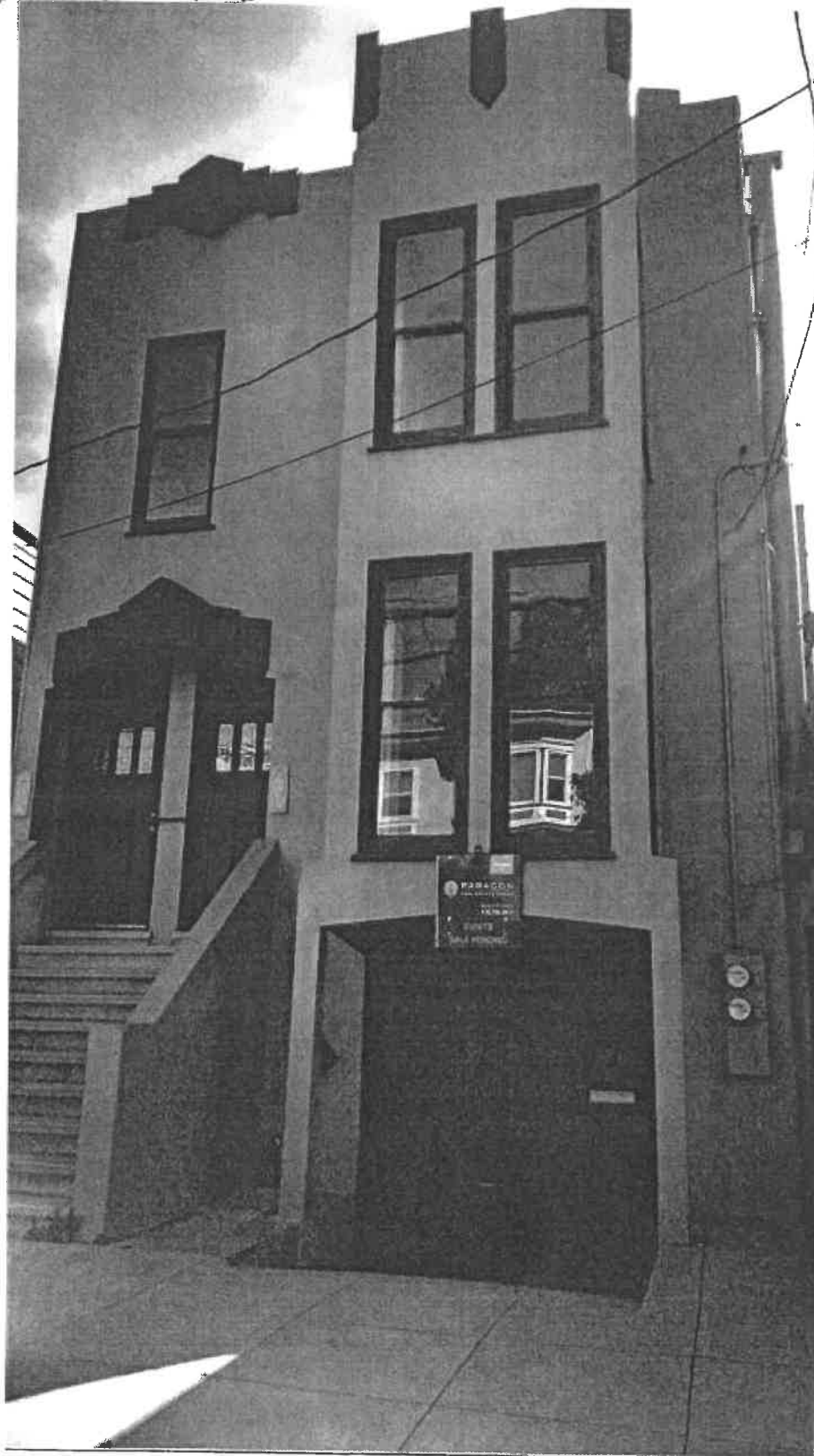
Primary façade, 1369-1371 Sanchez Street.
