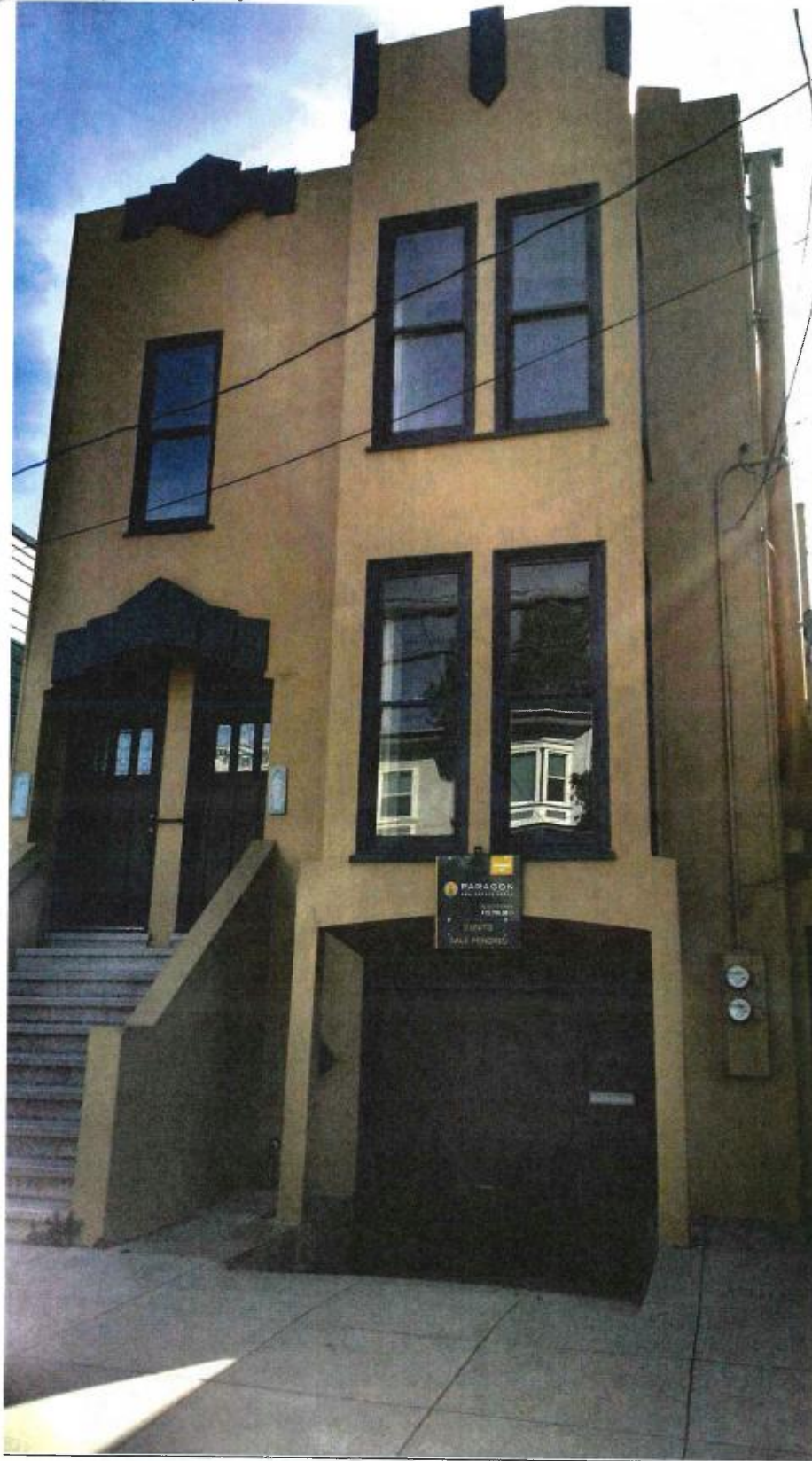
Primary façade, 1369-1371 Sanchez Street.
