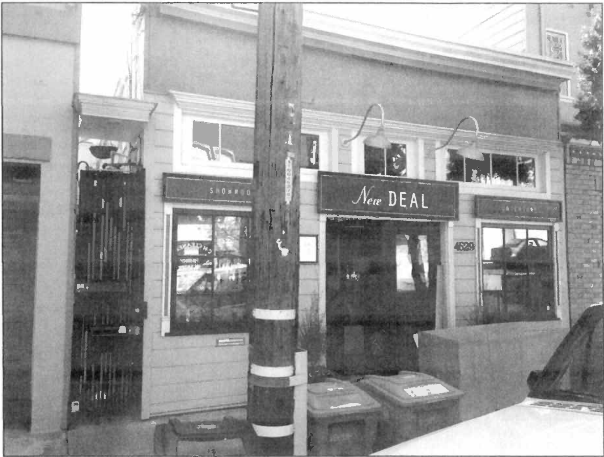
Figure 2: Subject building's front elevation, facing southwest
