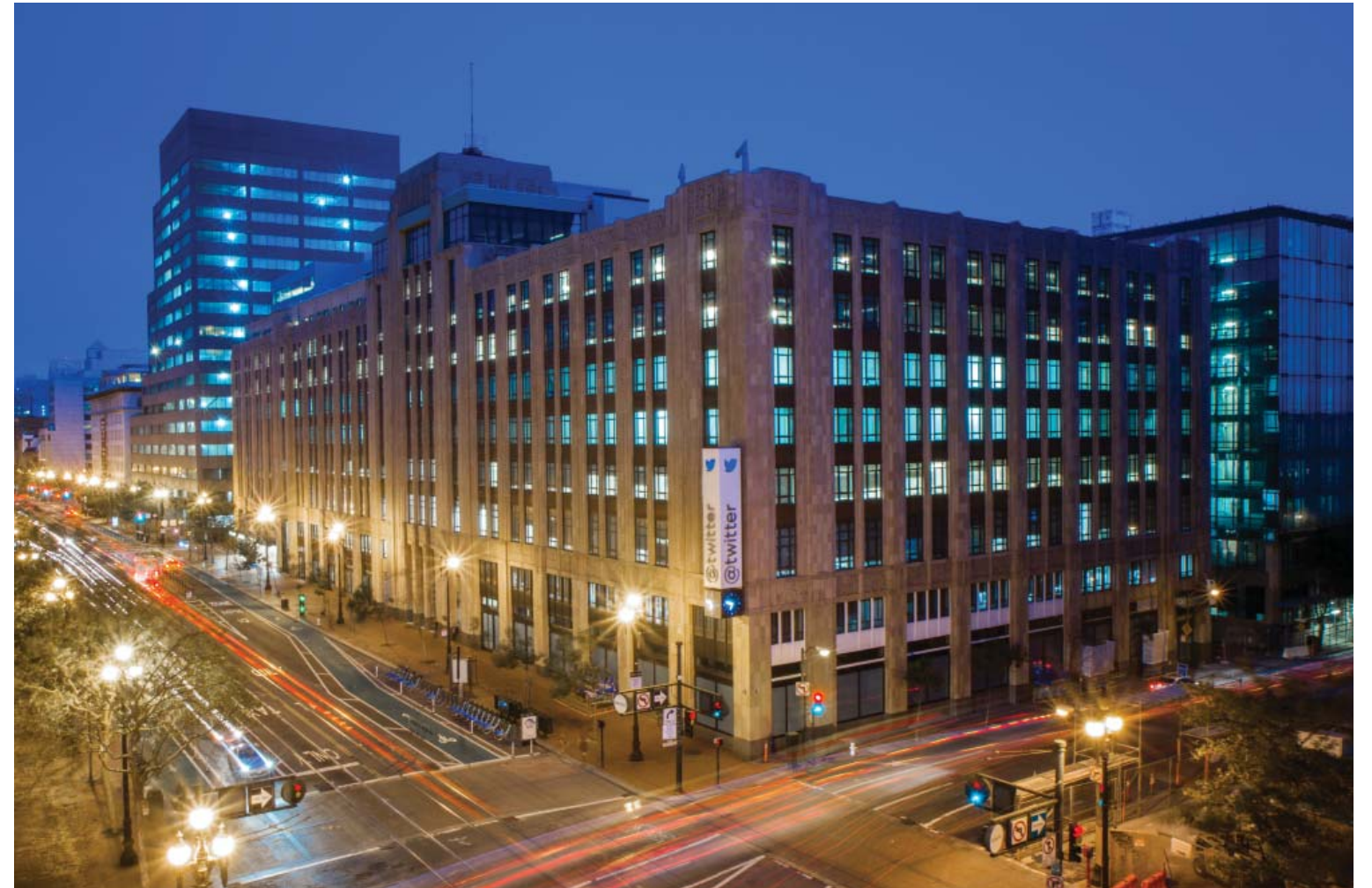
2. View looking east from Market Street.
