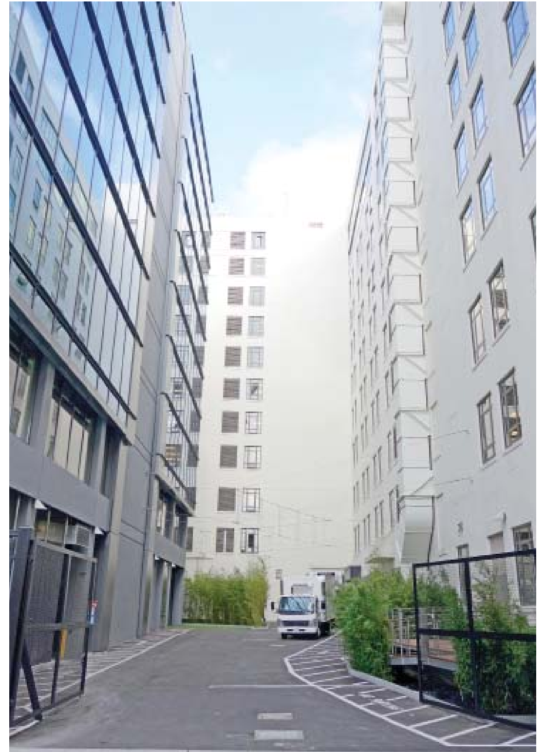
8. View looking north from Jessie Street towards Stevenson Street.
