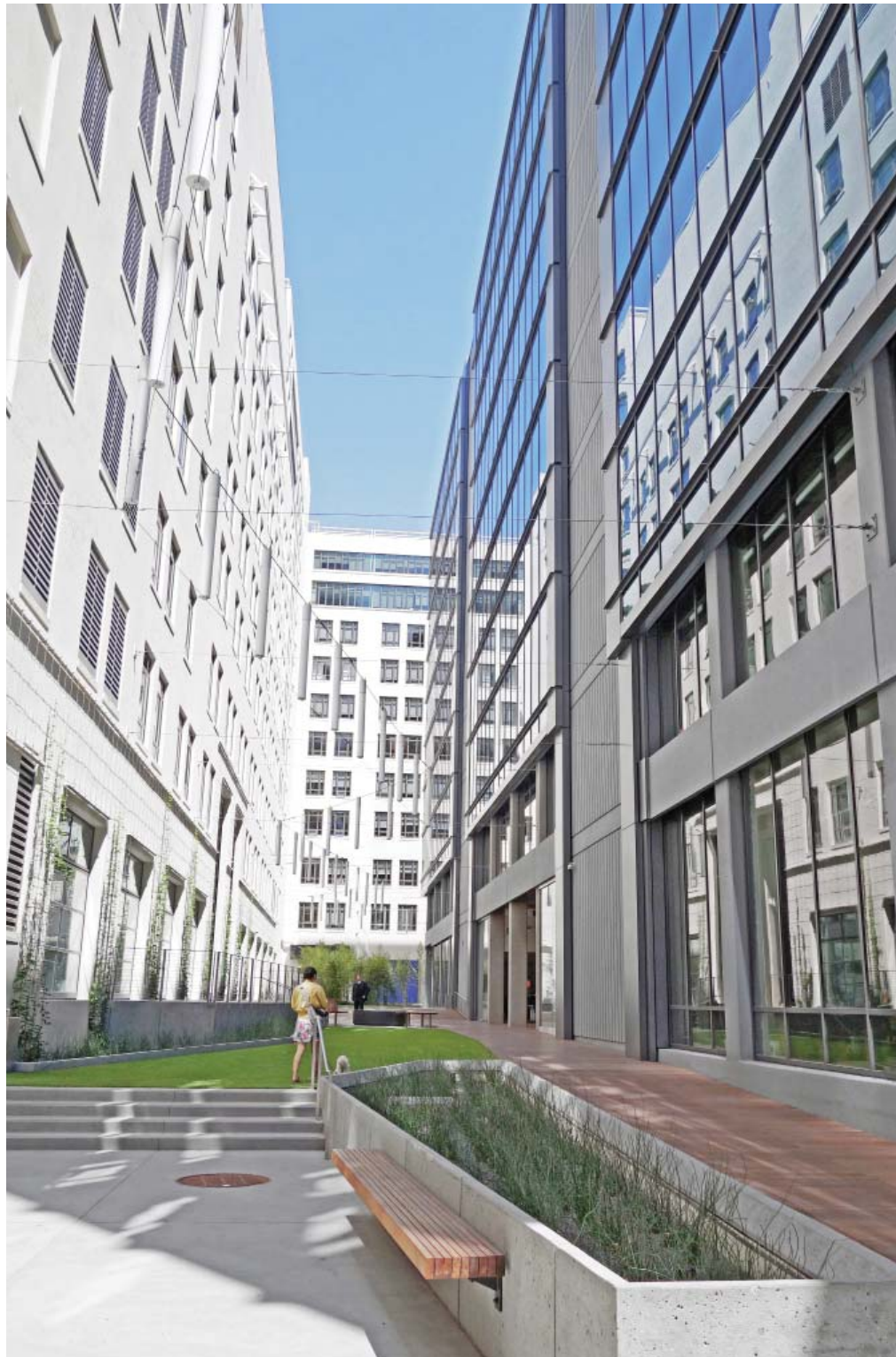
5. Stevenson street view looking east.
