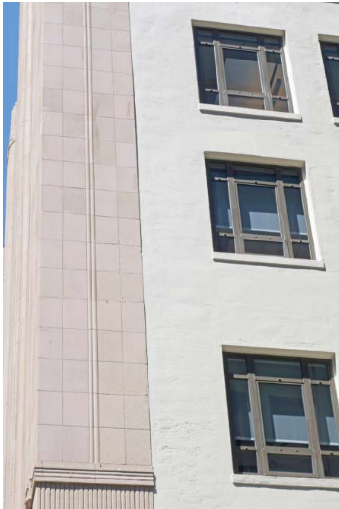
Detail view of 1355 Market Building rear (south) facade.
