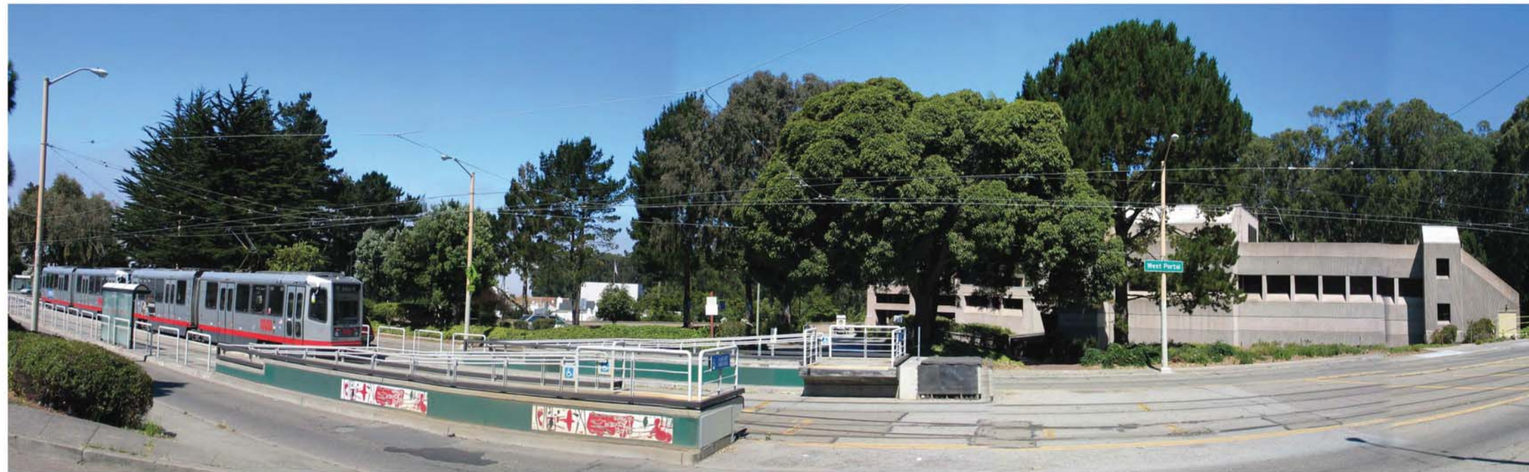
EXISTING SITE FROM WEST PORTAL
