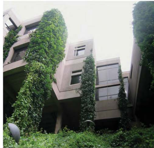
BELOW EXISTING BUILDING - PROPOSED LOWER LEVEL FUTURE CLASSROOM SPACE
