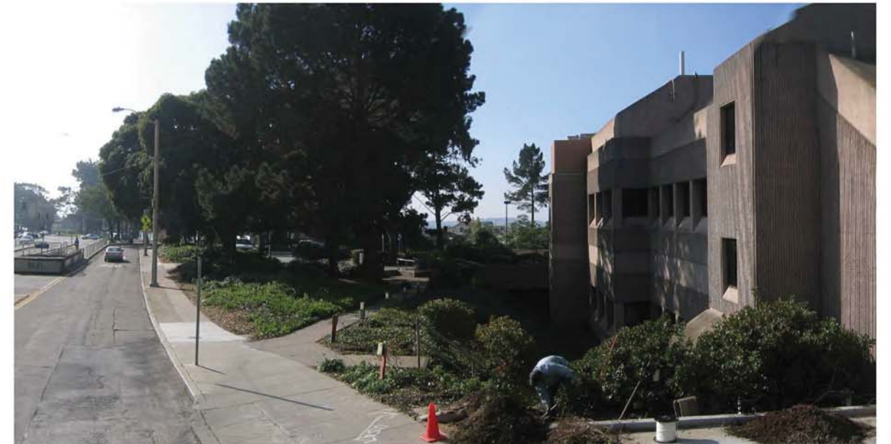
VIEW FROM WEST PORTAL AVENUE LOOKING SOUTH
