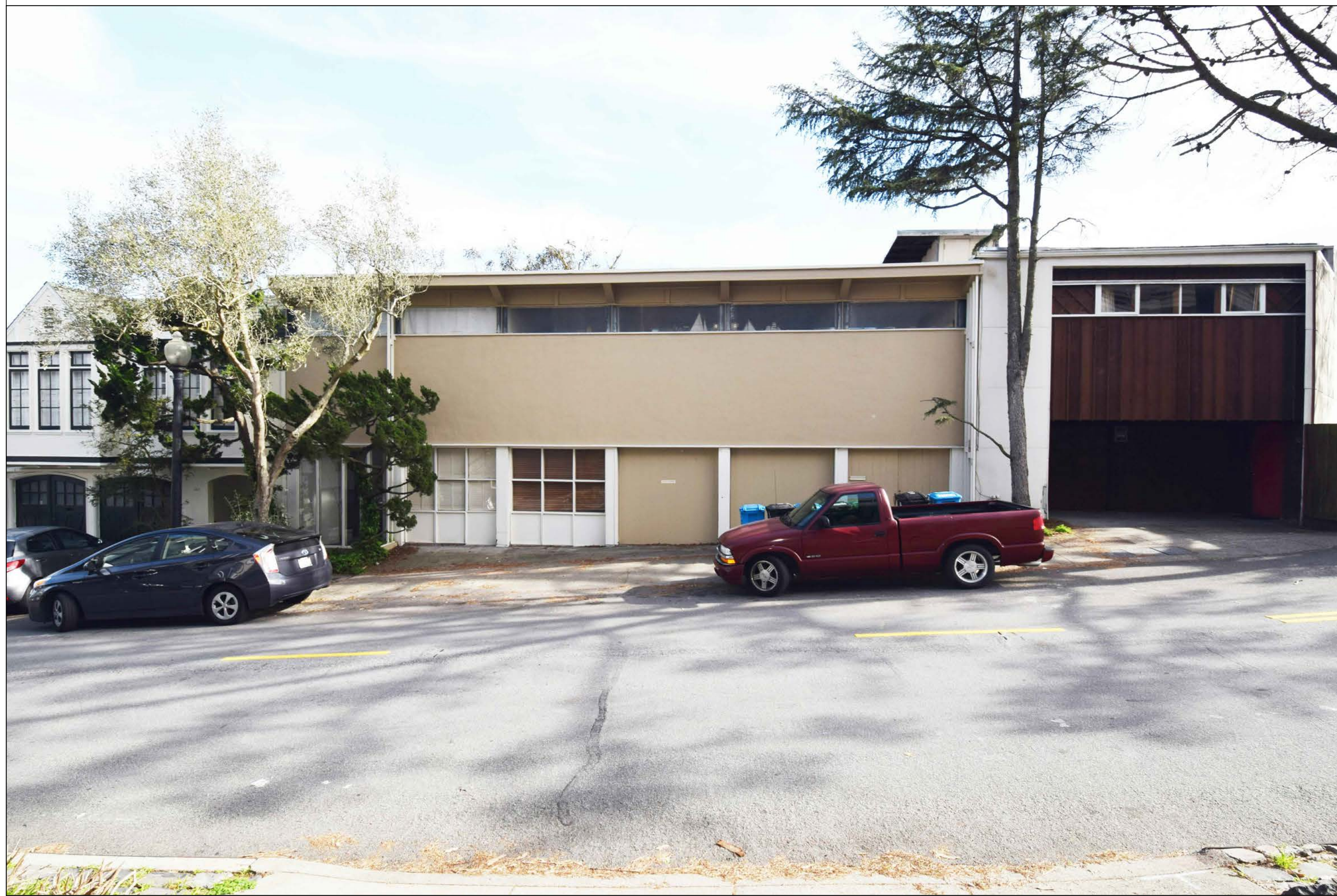
PHOTO LOOKING SOUTH @ UPPER TERRACE - EXISTING
