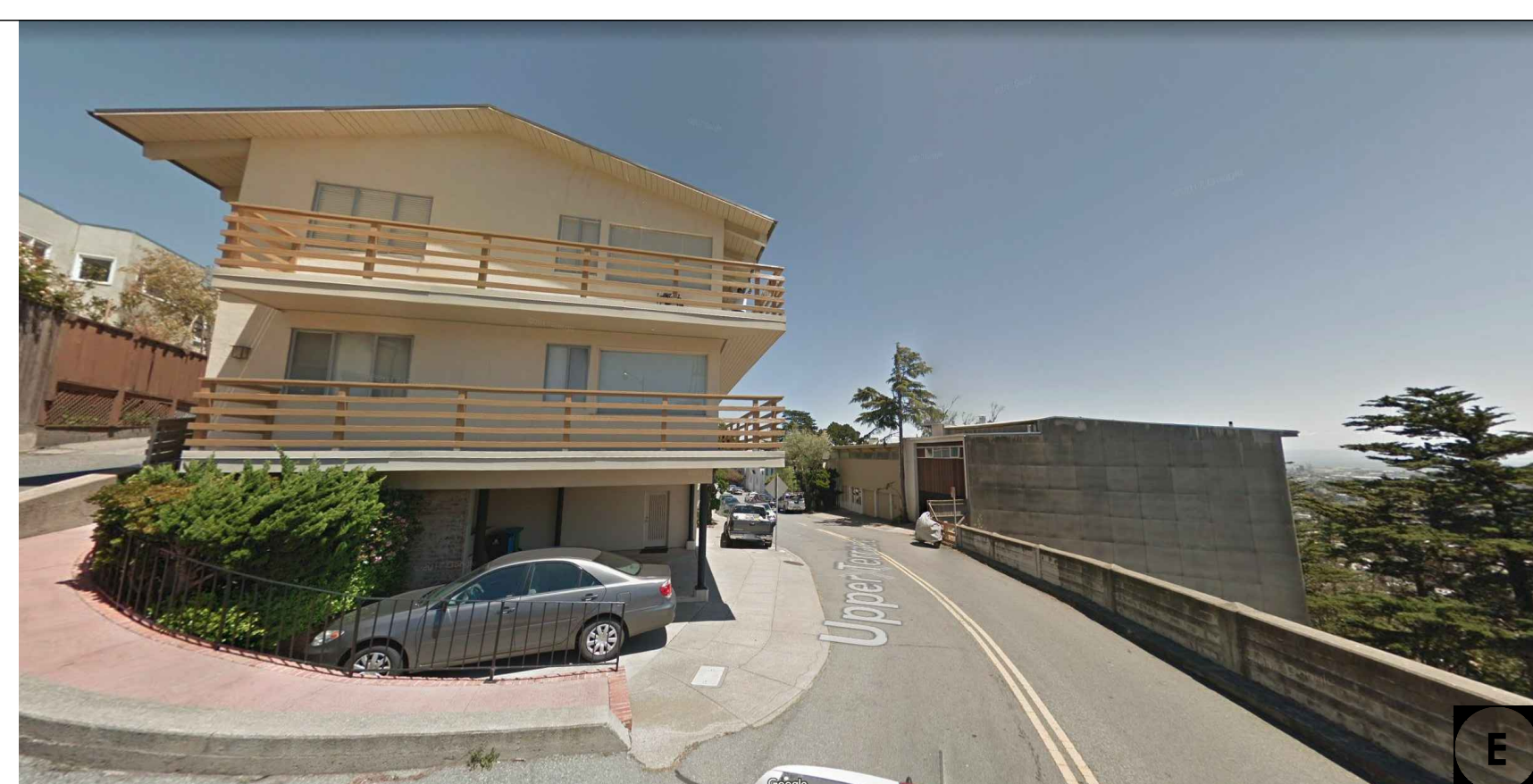
EAST ON UPPER TERRACE
