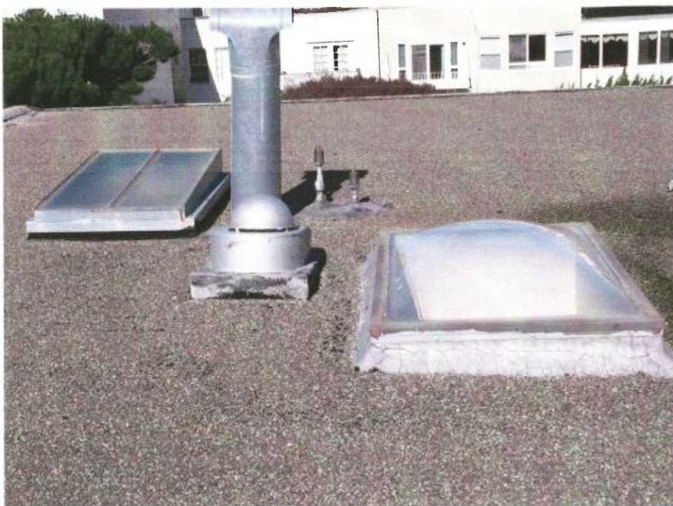
Skylights on neighbors roof to the East
