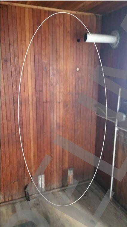
Photo # 22: Missing water heater.
