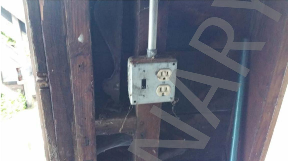
Photo # 39: Broken and improperly installed electrical throughout.
