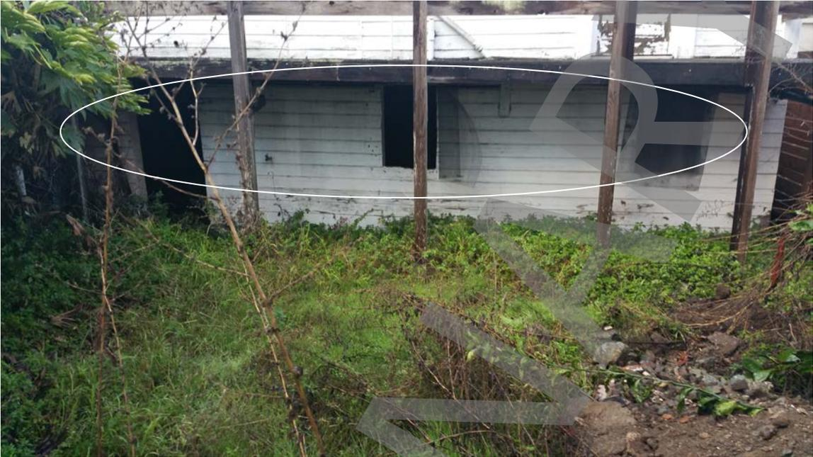
Photo # 23: Missing and broken windows and doors.
