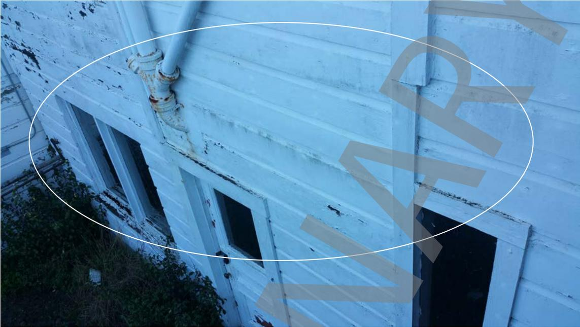
Photo # 14: Improper flashing, improper waterproofing detailing, rot, peeling lead paint at the back of the house.
