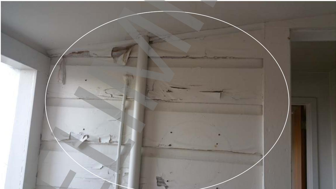
Photo # 13: Excessive moisture, rot, leaking, at mud room.
