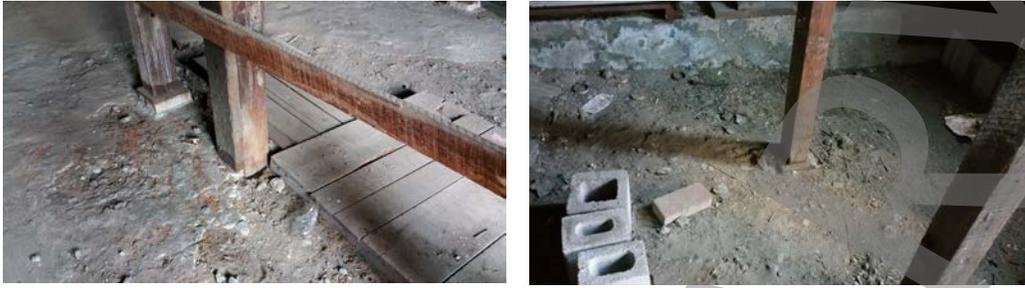
Photo # 35: Improper wood separation in area without weather protection, beetle infestation, rot.
