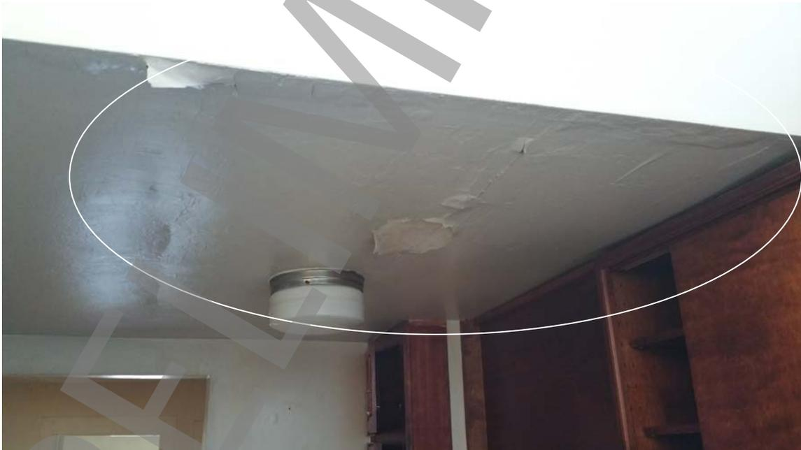
Photo # 9: Water damage to ceiling and electrical fixtures.
