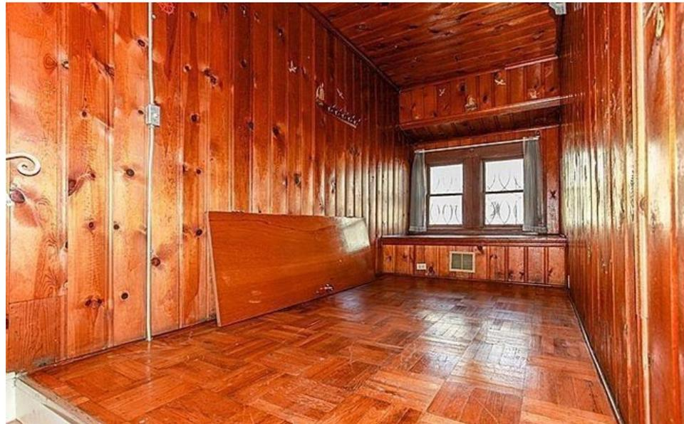
**Photo 6: This photo shows the room over the driveway. This room is elevated above the rest of the floor area because it was created by filling in the area over the driveway at a level that would have still allowed a car to access the space below.**
