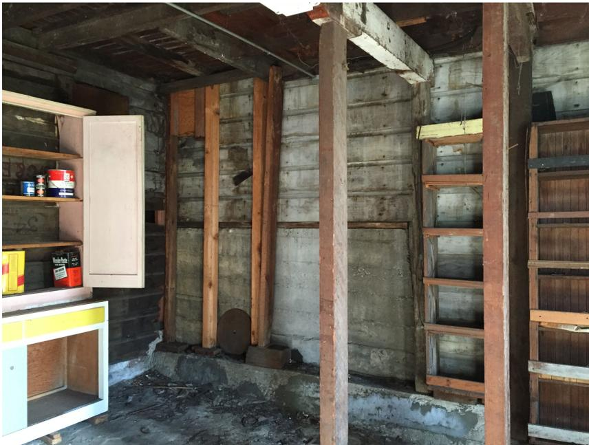
**Photo 20:** this photo shows the area to the left of the previous photo. Note the funky posts, propped up on blocks, supporting the corner of the addition. Again, this is a completely unorthodox method of construction.
