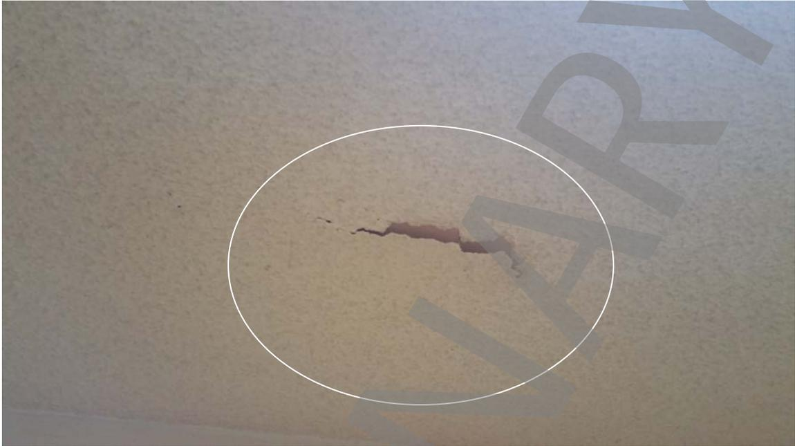
Photo # 12: Flaking and peeling asbestos finish in dining room.
