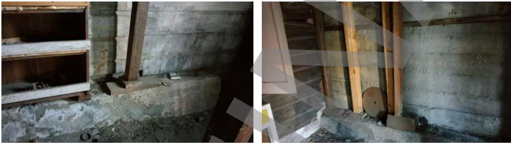
Photo # 36: Homemade, unsafe built very out of plumb posts on improper foundation, typical.
