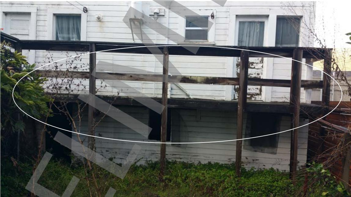
Photo # 24: Rotten walkway and peeling lead paint.
