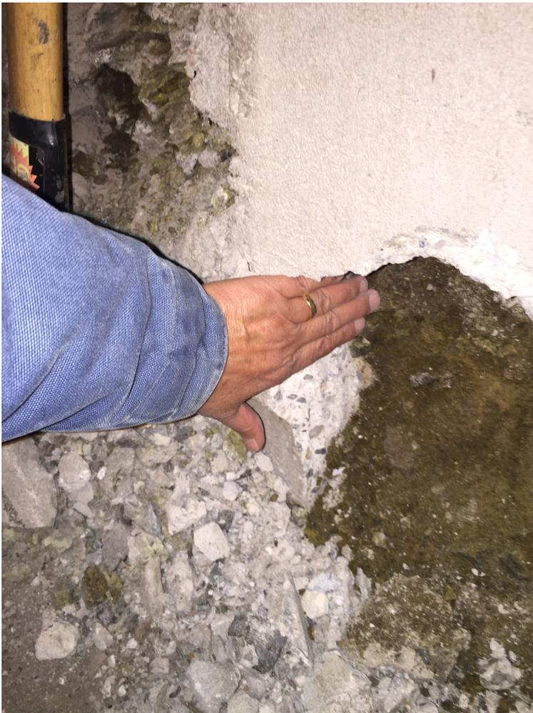
**Photos 3 & 4: In these photos I use my hand as a reference to demonstrate the depth of the door patch. Note that the depth of the patch is roughly the depth of my fingers at the top of the patch, and also that it is the same depth below where the soil is exposed. This indicates that the original retaining wall did not extend down to the bottom of the current floor level, and that it was undermined with the secondary excavation.**
