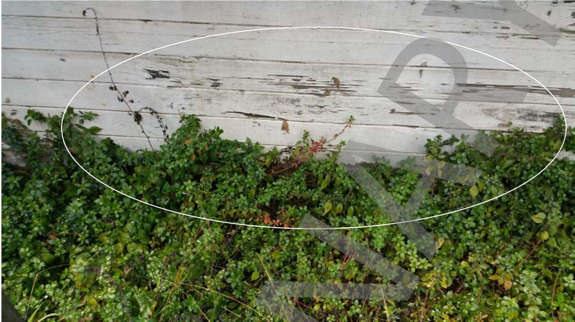
Photo # 25: Rotten siding causing peeling lead paint.
