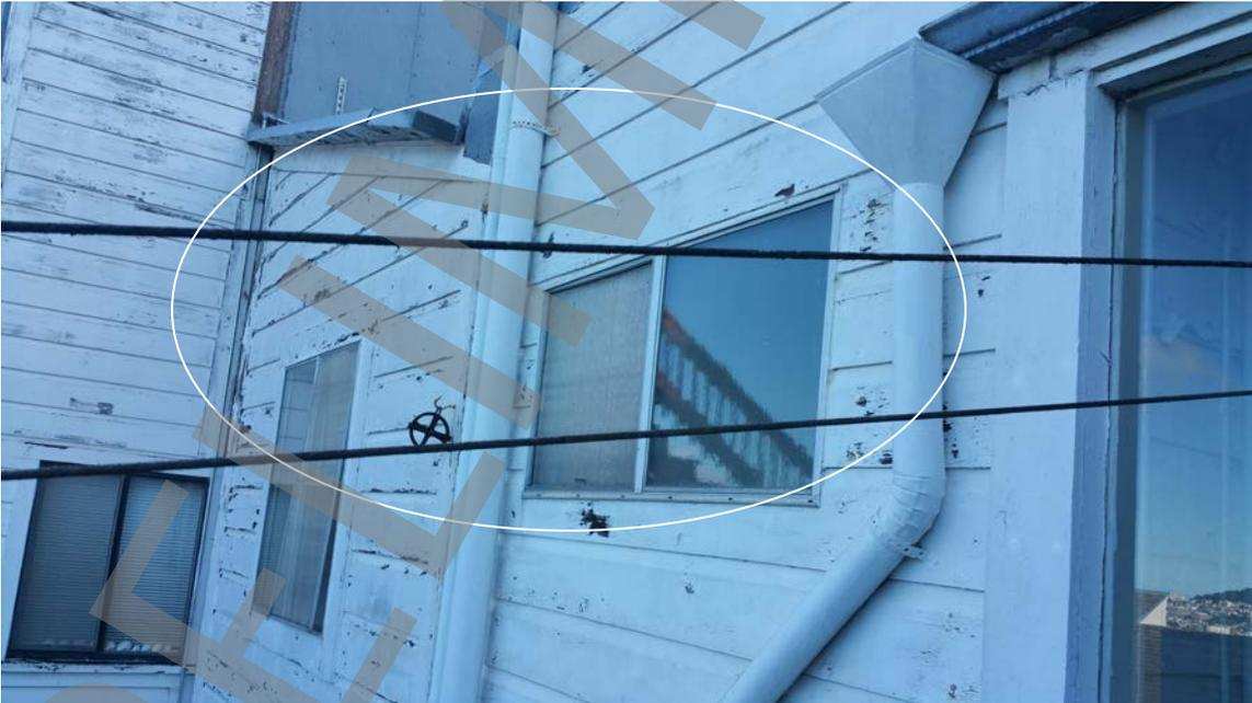
Photo # 15: Improper waterproofing and flashing. No trim.
