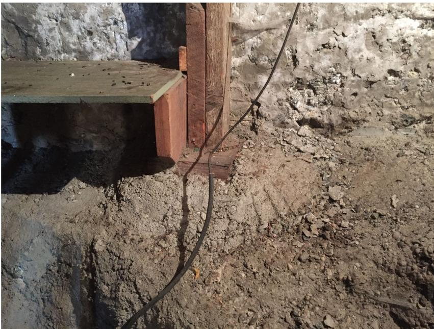
**Photo 7: This photo shows a post supporting the central bearing line adjacent to the front retaining wall. Note how the support at the base of this post has been built up with concrete on the surface of the excavated face. This suggests that the original support for this post was also undermined through the process of the secondary excavation.**
