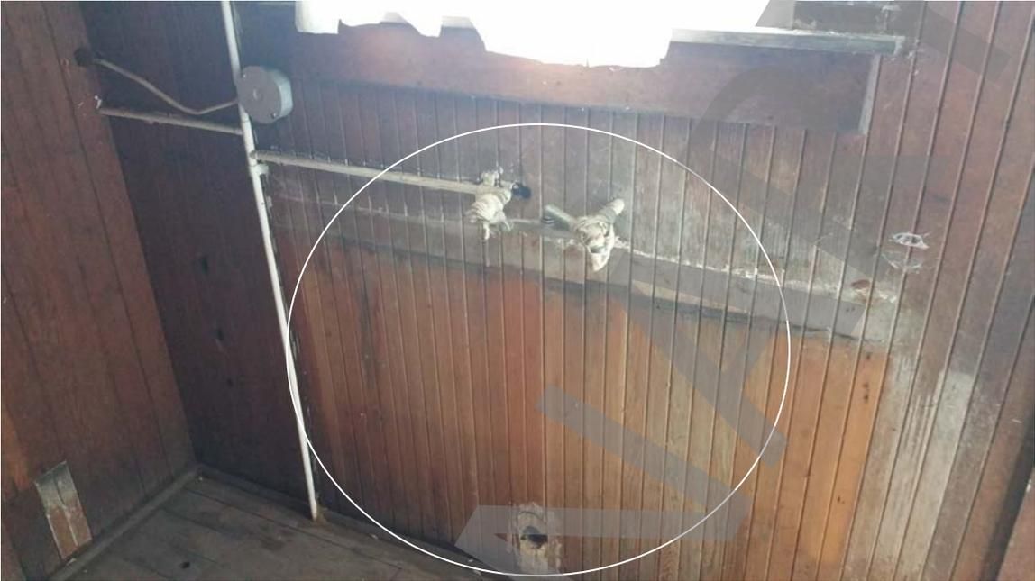
Photo # 21: Missing sink and drain.
