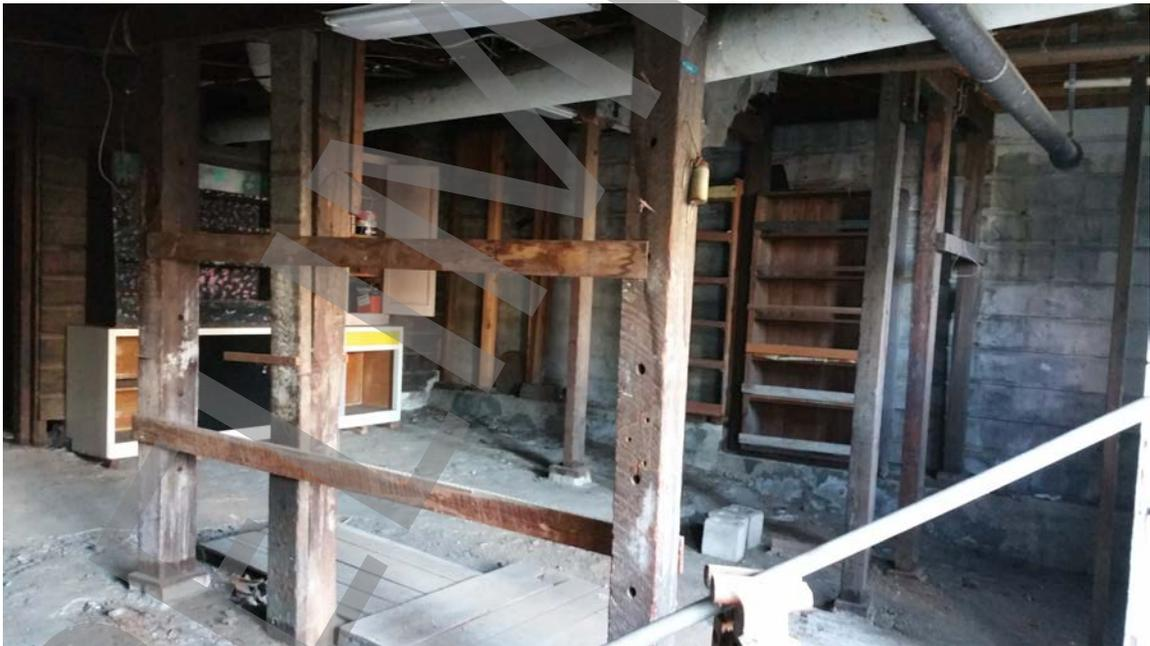
Photo # 40: Maze of homemade-design posts and beams, unable to carry required loads, throughout. Undersized joists and beams, throughout.
