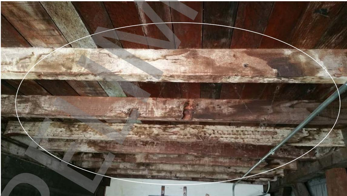
Photo # 42: Undersized floor joists, typical.
