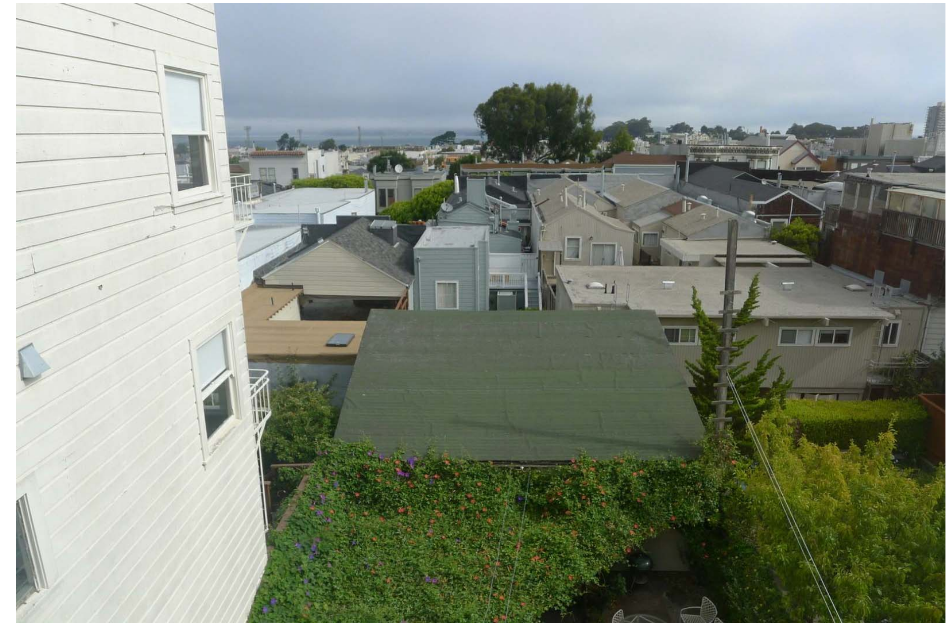
VIEW FROM 2ND FLOOR AT REAR YARD
