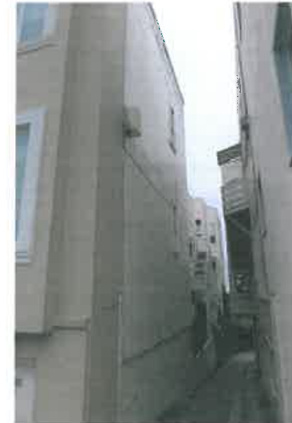
ADJACENT NEIGHBOR - PROPERTY LINE WINDOWS
