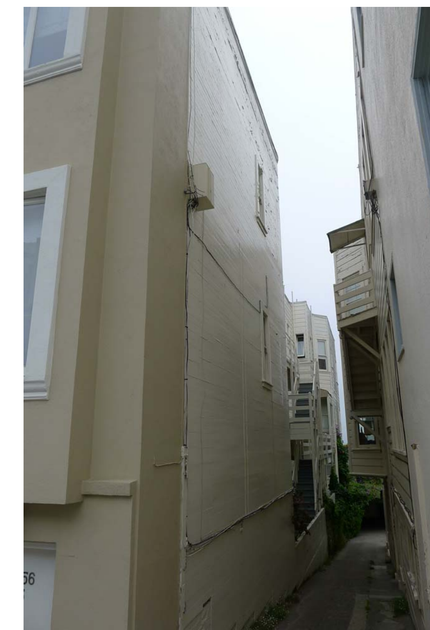
ADJACENT NEIGHBOR - PROPERTY LINE WINDOWS
