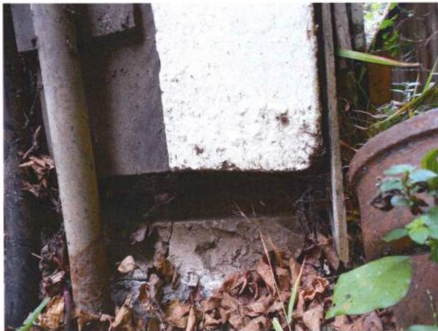
Photo 20: This is the corner of the building at the front showing another view of the improper grade condition and the exposed sill plate.
