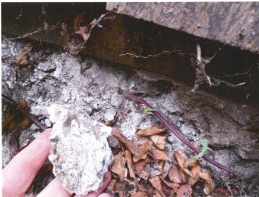
Photo 18: This photo was taken outside at the front of the building. Note the chunk of concrete that has crumbled away. Also note that the sill plate is too close to the soil and is completely exposed, which will allow water to saturate it and lead to rot over time.
