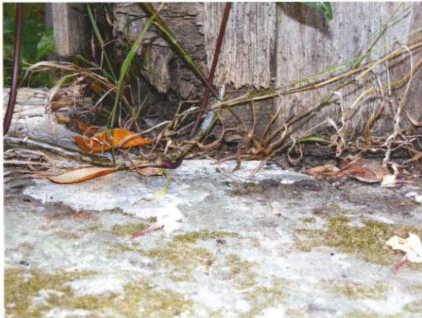
Photo 24: This is a close up of the previous photo. It shows how the framing gets saturated and rots over time due to continual exposure to moisture.
