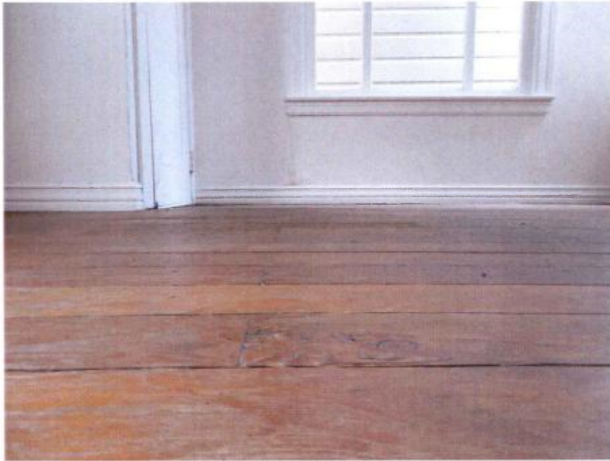
Photo 27: This photo shows the floor at the main entrance. Although the slope of floor is actually quite pronounced, the photo does show some of the slope. This is a considerable differential for such a short distance.
