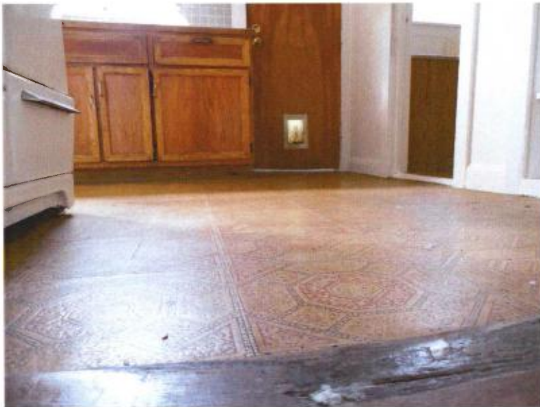
Photo 30: This photo shows the effect of settlement at the back of the building. Again, the photo does convey the true extent of the settlement, but like the front addition, it is quite pronounced when you actually stand in the house.
