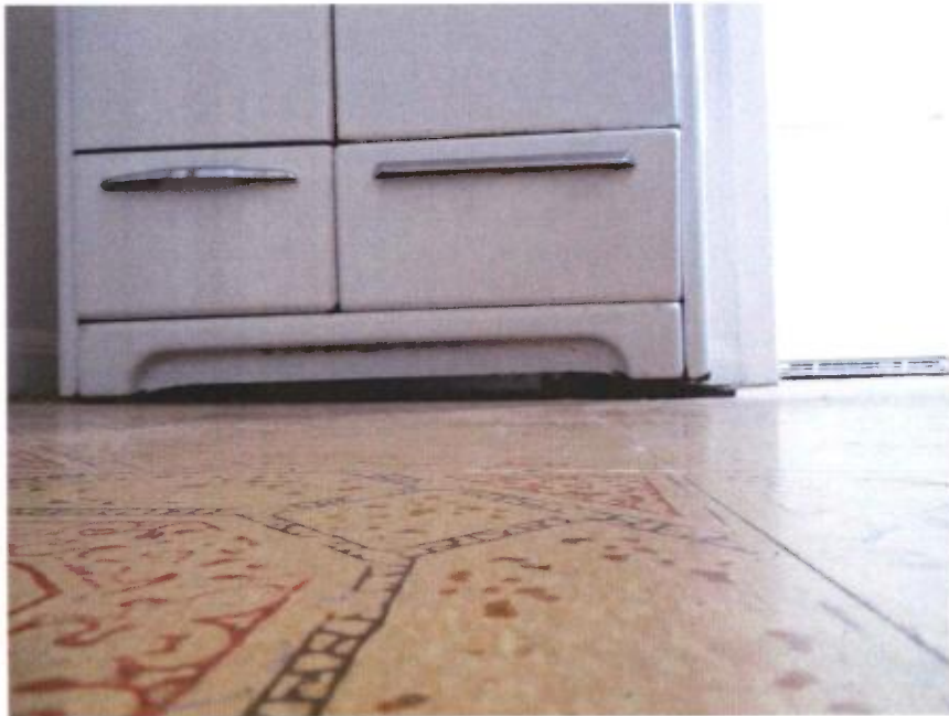
Photo 31: This photo shows that the stove has been shimmed at its base to compensate for the floor sloping so significantly towards the back of the building. Again, consider that the stove is only about 3-feet wide, so this is a considerable slope over such a short distance.
