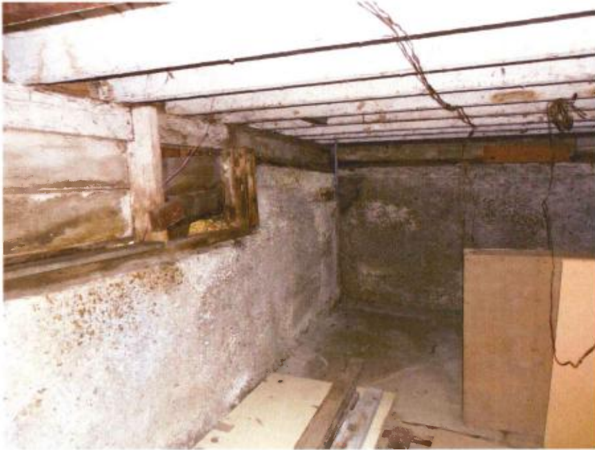
Photo 15: This photo shows the left rear corner of the storage area. Note the rotten framing at the left, which is due to improper grade. The foundation shows signs of spalling throughout.
