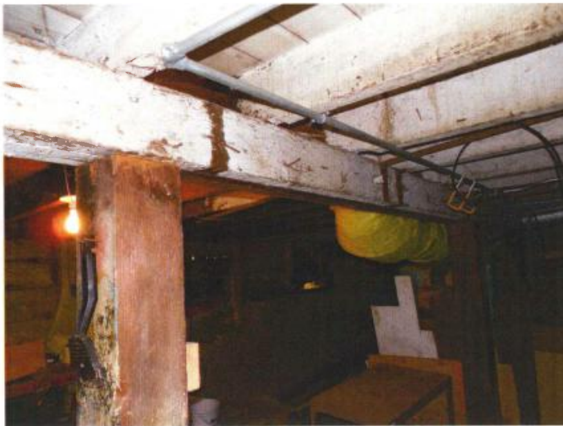
Photo 12: A built-up beam supports the floor at the mid span of the joists, the bearing wall above, and the ceiling joists at their mid span. It is comprised of three 2x6 members sandwiched together. This beam does not meet the code in effect at the time of original construction and needs to be upgraded.
