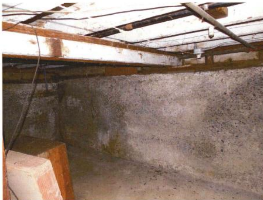
Photo 16: This photo shows the center of the retaining wall at the back of the storage area. The centerline support beam terminates at the top of this wall, and its proximity to the exterior grade has also led to some decay in the end of this member.
