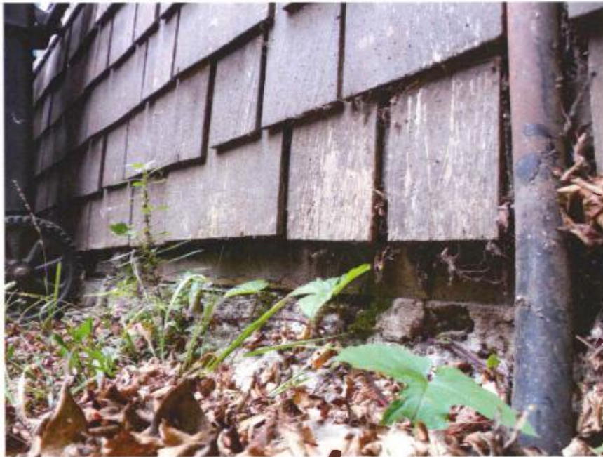
Photo 19: This is another view of the sill plate across the front of the building. The siding should always extend below the bottom of the sill plate to protect it from the elements, but in this case the plate is too close to the ground to extend the siding without burring it in the dirt.
