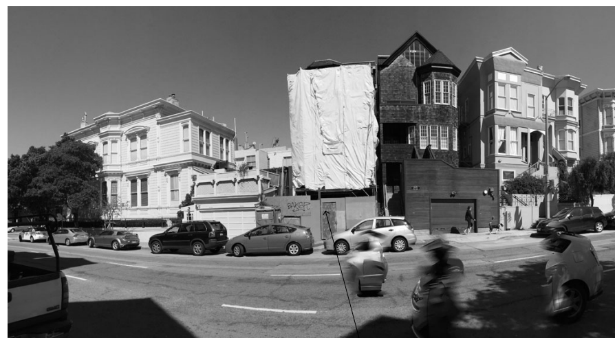
4 STREET VIEW- PANORAMIC —2178 PINE STREET
