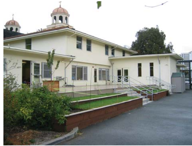
EXISTING ELEMENTARY SCHOOL BUILDING NTS 4
