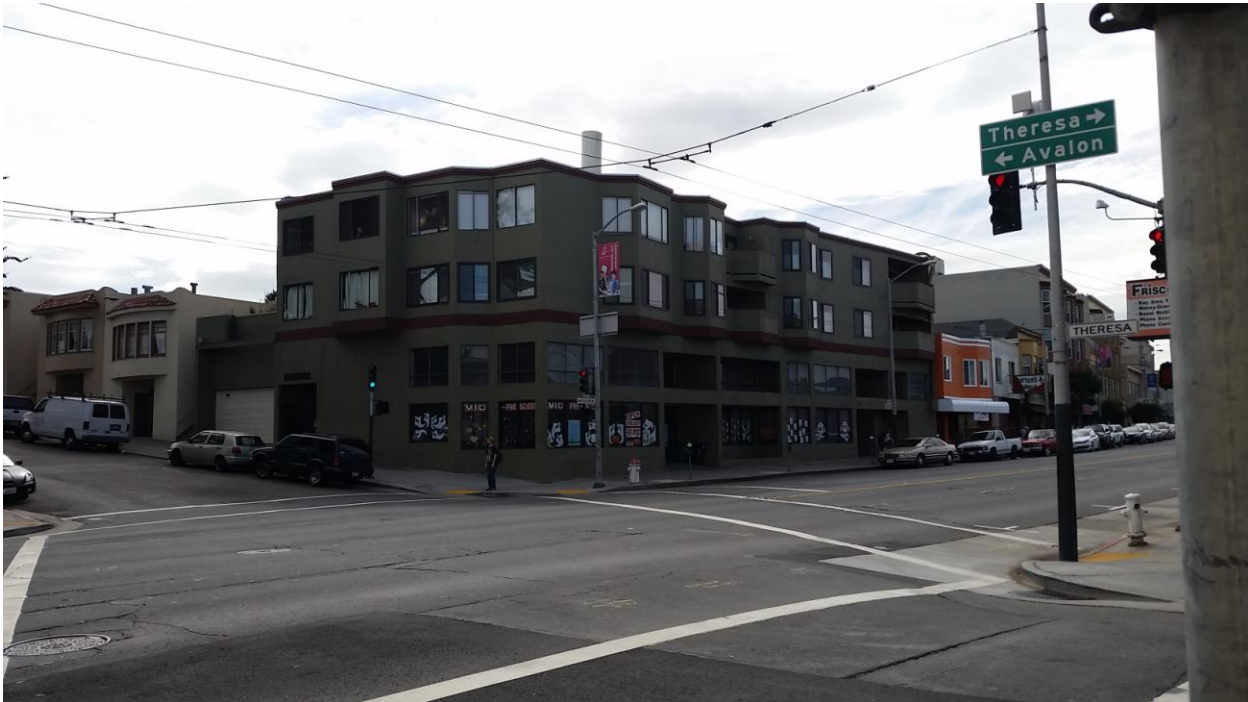
View of site looking east along Avalon Ave.
