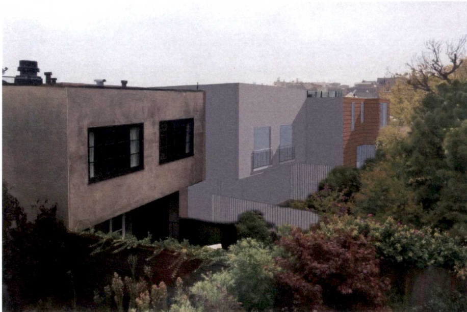
From 2nd level, Kitchen & Family room, 2750 Lyon St. EXISTING CONDITION
