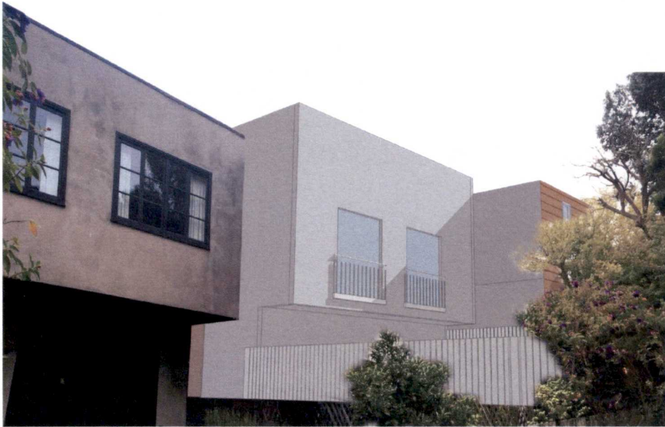
From Backyard, 2857 Filbert EXISTING CONDITION
