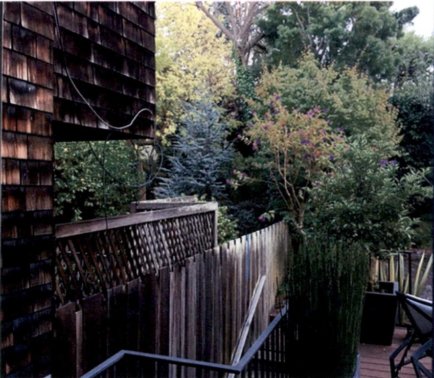
From Dining Room, 2857 Filbert EXISTING CONDITION
