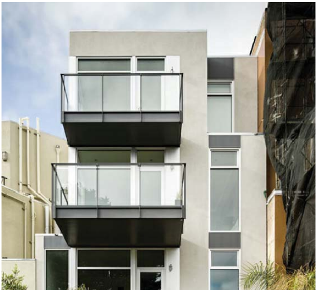
RAILING: 1/2" x 2" STAINLESS STEEL FLAT BAR RAILING AND 2" x 2" POSTS WITH TEMPERED GLASS (ALTERNATE: POWDER COAT TO MATCH WINDOW & DOOR COLOR)
