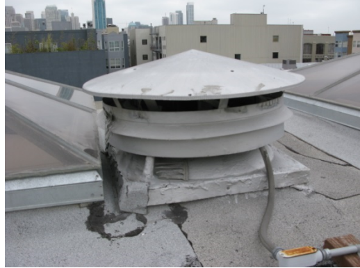
Typical skylight vent
