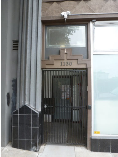
Non-original metal security gate and aluminum storefront door in vestibule
