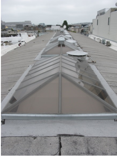
Row of skylights
