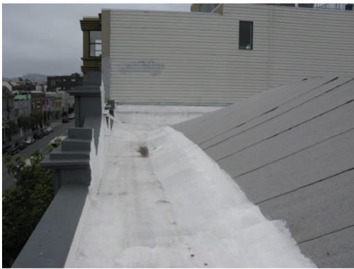
Coating (elastomeric?) at roof perimeter gutters
