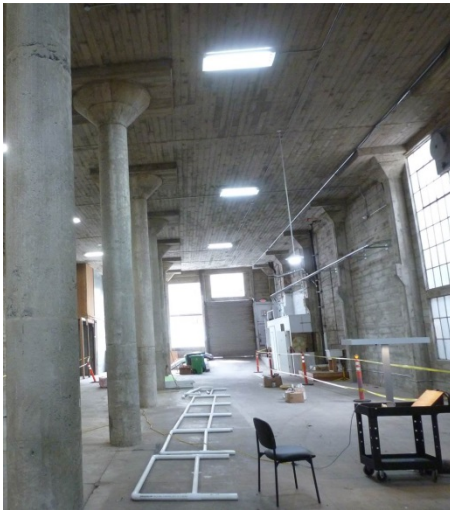
Concrete columns and board formed concrete; wood floor and board formed ceiling at Mezzanine.
