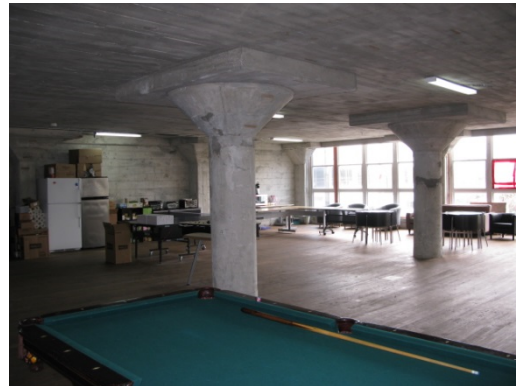
Concrete columns and board formed concrete; wood floor and board formed ceiling at Mezzanine.
