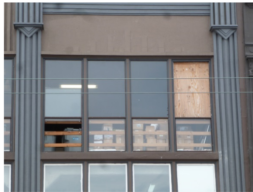
Vertical rectangular projecting ornamentation on the face of the band between the pilasters has been painted over and is obscured
