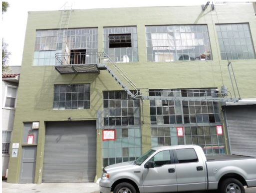
Metal fire escape at Natoma facade
