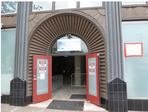
Main entrance doors are non-original and in good condition
