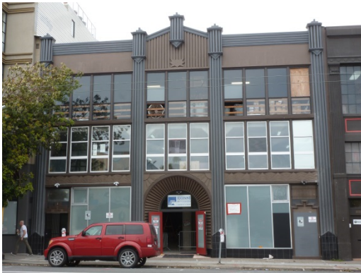
Howard Street windows-aluminum replacements
