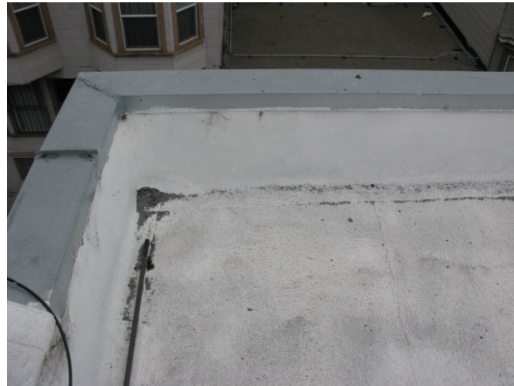
Typical low, un-braced parapet with metal coping
