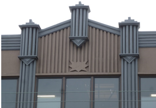
Detail of fluted column, triangular parapet and star medallion
