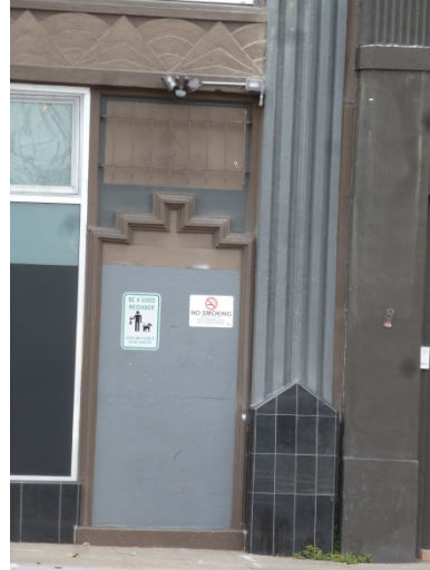
Original door frame and transom frame
