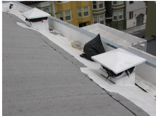
Typical mechanical penetrations
