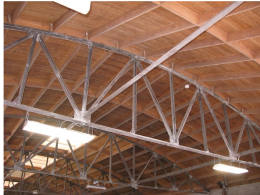
Exposed roof framing structure
