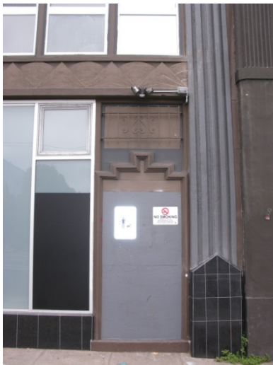
Black granite tile column bases and storefront bulkhead
