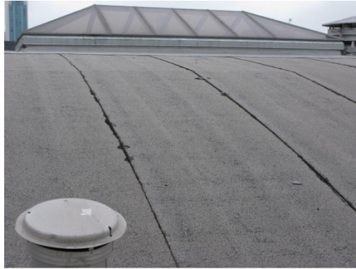
Detail of membrane installation
