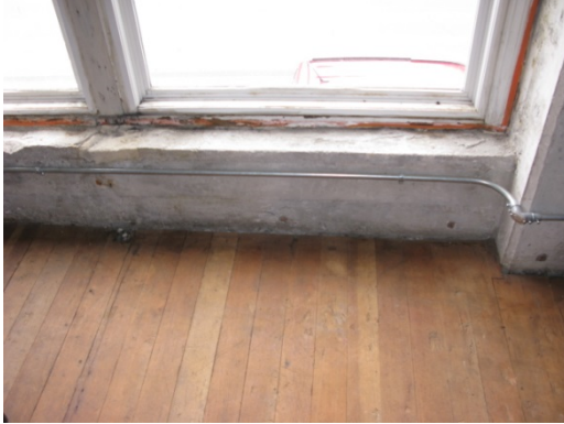
Wood sills and frames at Howard Street
